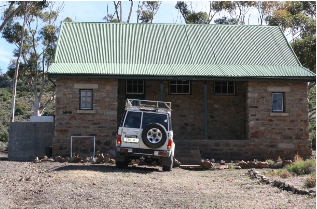
Figure 9: Old School building
