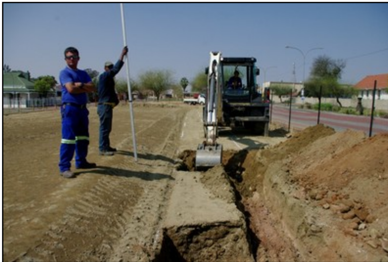
Plate 6: Mechanical trenching – southern structure foundations [2]
