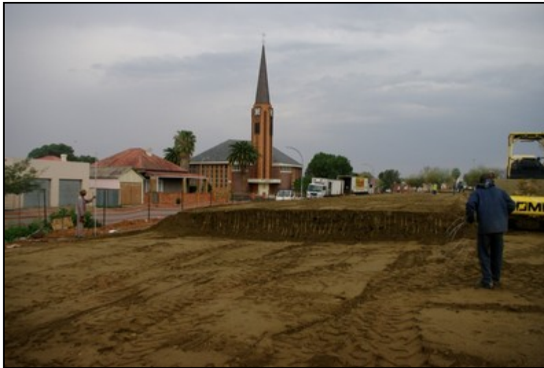
Plate 1: Final site measurements prior to mechanical trench foundation excavations
