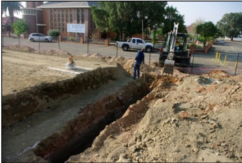
Plate 10: Mechanical trenching – eastern structure foundations
