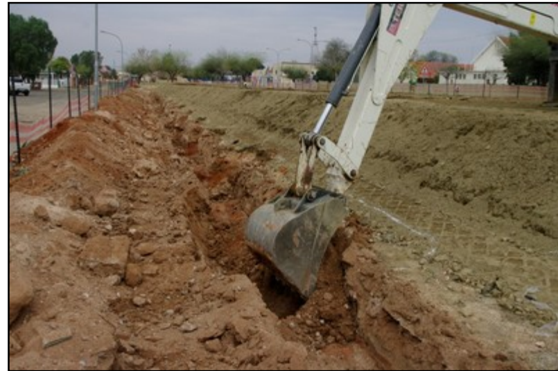
Plate 3: Mechanical trenching – northern structure foundations [2]
