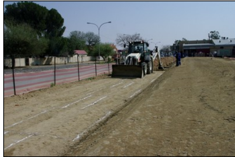
Plate 7: Foundation demarcation and trench excavation, southern structure foundations
