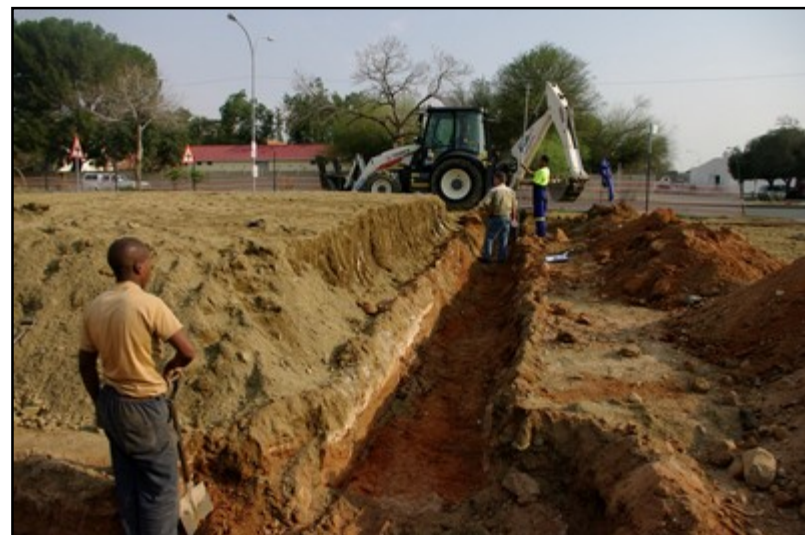
Plate 4: Mechanical trenching – western structure foundations
