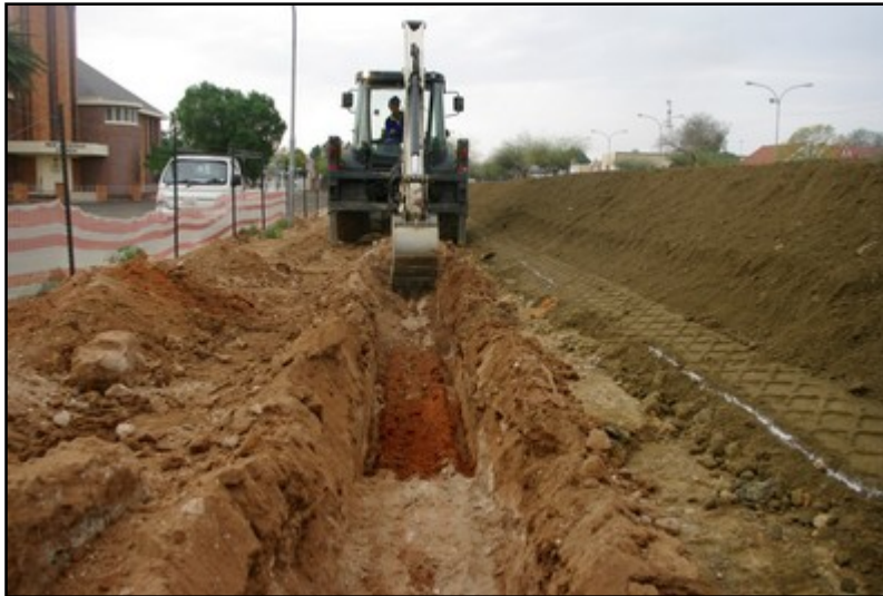
Plate 2: Mechanical trenching – northern structure foundations [1]
