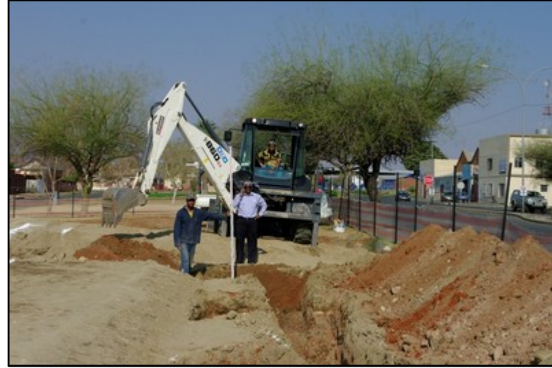
Plate 8: Trench excavations along the south-eastern boundary of the site
