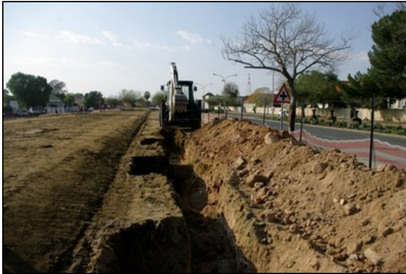
Plate 5: Mechanical trenching – southern structure foundations [1]
