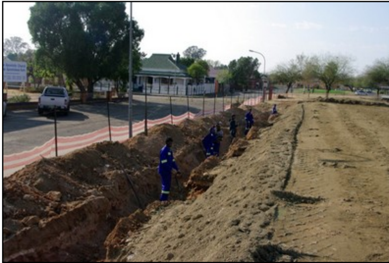
Plate 9: Manual cleaning of mechanically excavated foundation trenches
