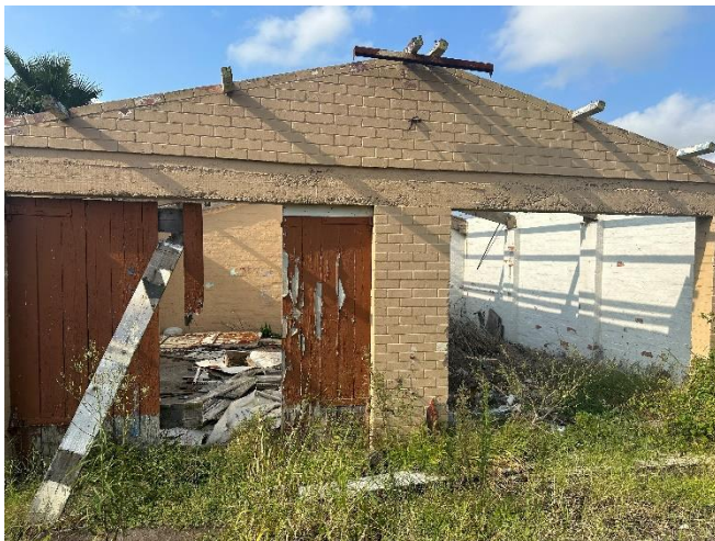
THE ROOF WAS STRIPPED BY VAGRANTS AND SOLD. THE STRUCTURE IS EXPOSED TO THE SKY.
