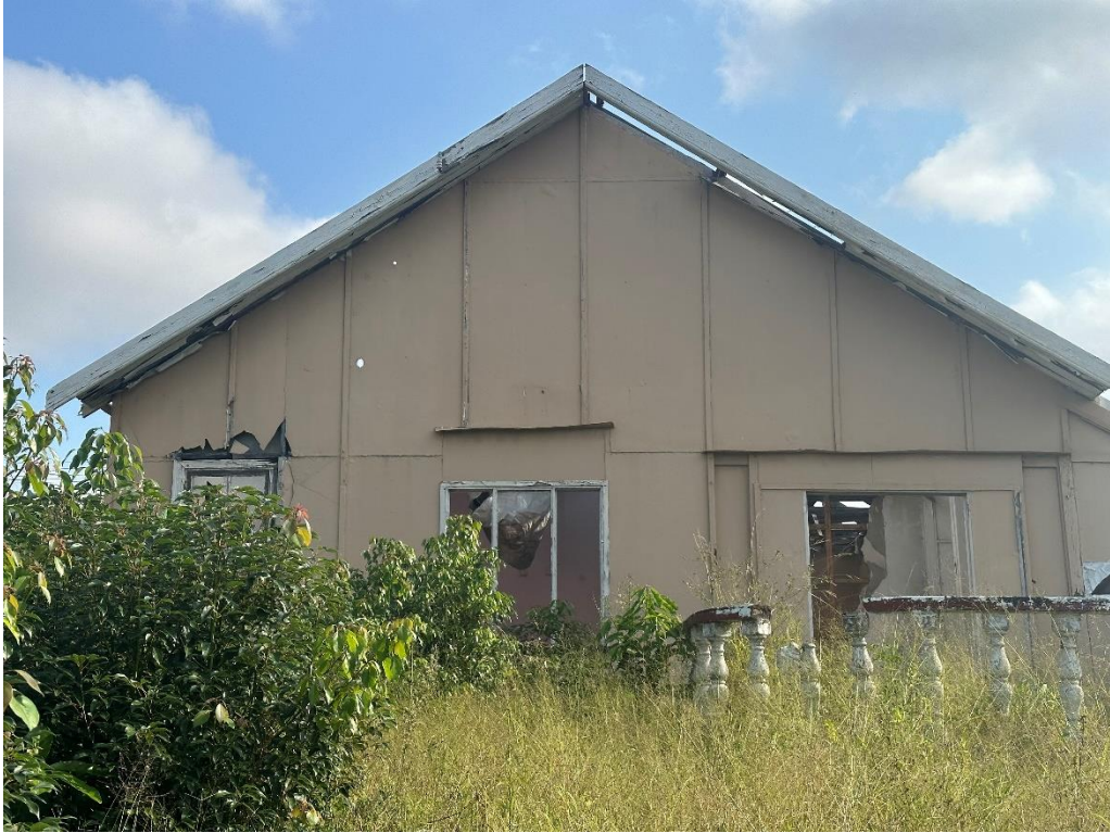
NORTH-EAST ELEVATION OF REAR OF MAIN DWELLING.
