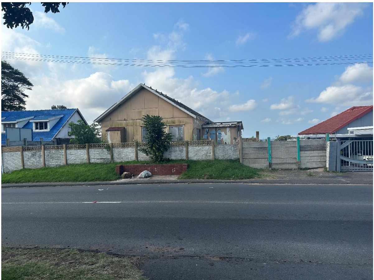
FRONT ELEVATION FROM FREMANTLE ROAD– SOUTH-WEST ELEVATION
