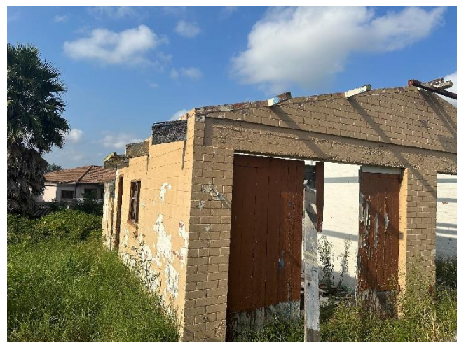
THE ROOF WAS STRIPPED BY VAGRANTS AND SOLD. THE STRUCTURE IS EXPOSED TO THE SKY.
