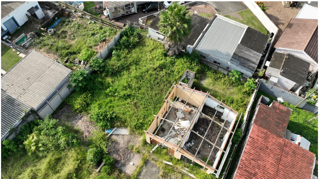
AERIAL VIEW OF 5 FREMANTLE ROAD (OUTBUILDING VIEW – NORTH-EAST ELEVATION)
