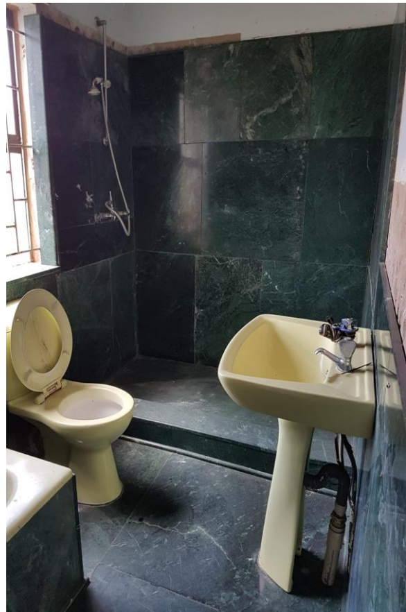
Image 05 – Existing Ground Floor Bathroom
