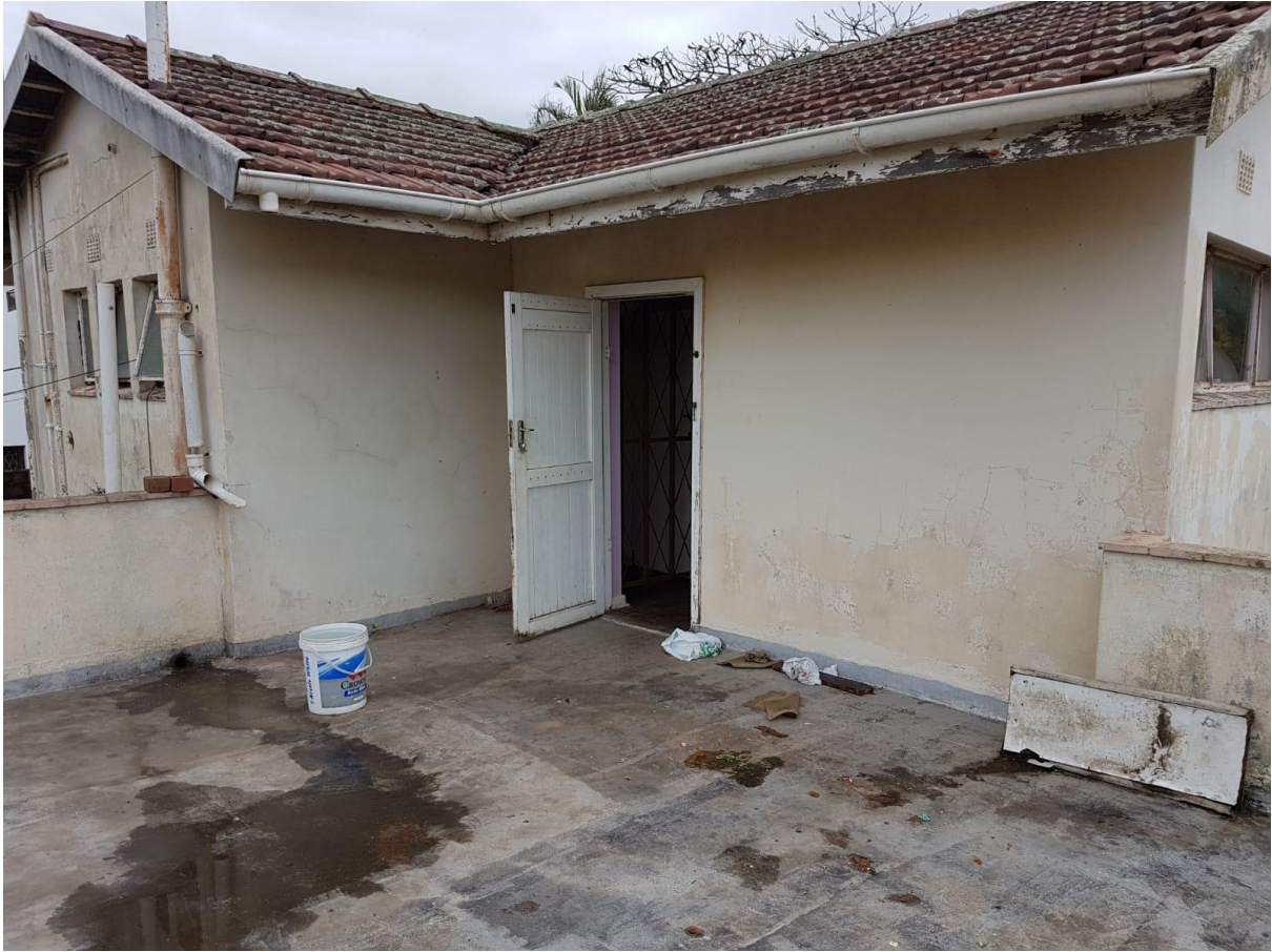
Image 07 – View of building from upper deck
