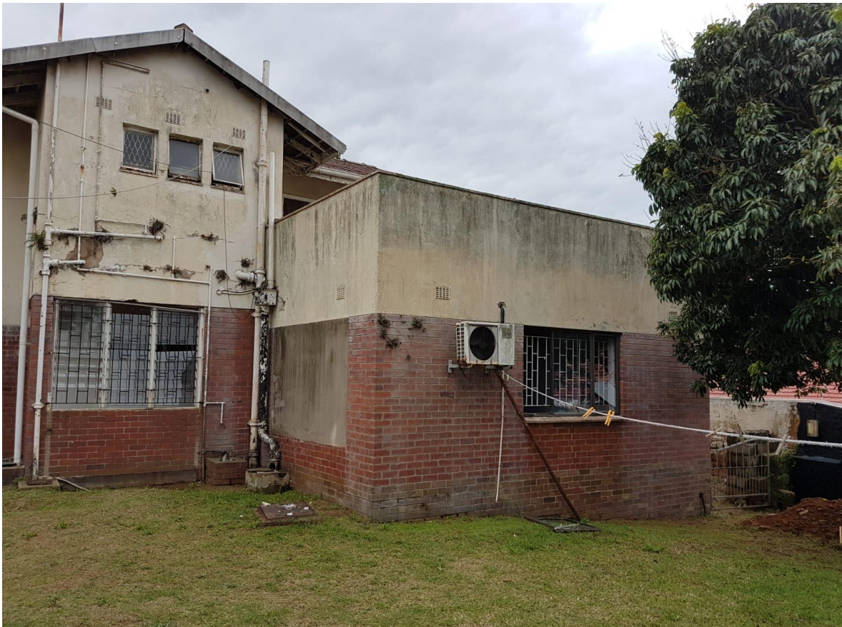
Image 06 – View of building from the rear.
