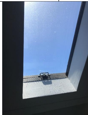
Loft bathroom skylight
