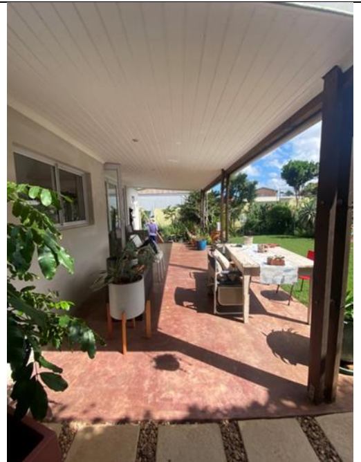
Veranda detail from the North
