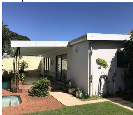
East Elevation – Outbuilding
