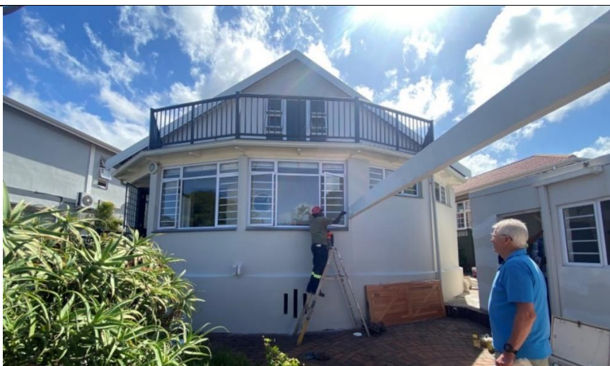
East Elevation from parking
