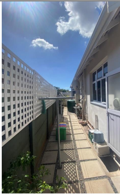
North elevation – west end / scullery
