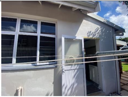
North elevation – south end
