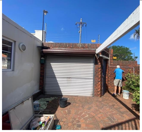
Garage door to parking – inside view
