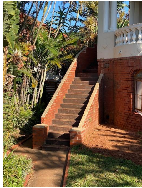
Entrance Stair from garden
