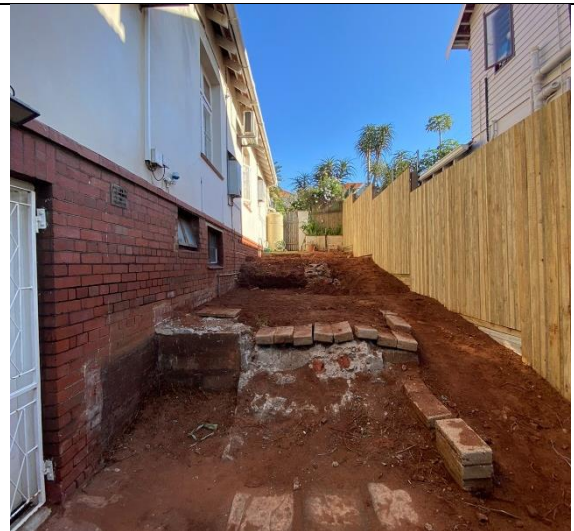
Garden Terrace and Ramp
