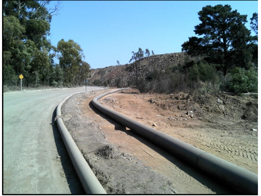
Figure 5: Pipeline located within the road reserve.
