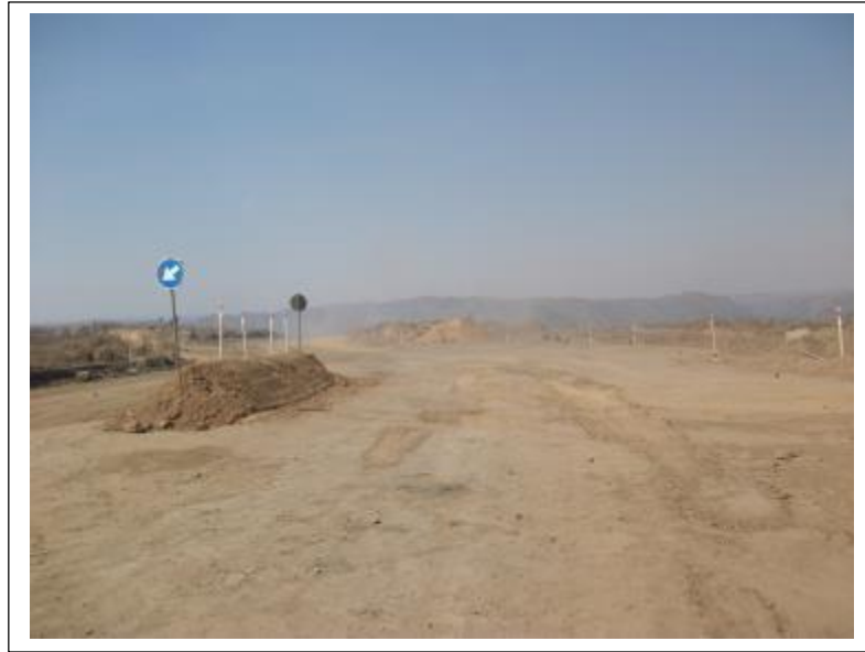
Figure 7- Existing haul roads, excavations, cleared surfaces and dumps of soil have disturbed the proposed Pit 2A extension area (which includes the location of the planned Pollution Control Dam and the haul road (above)).
