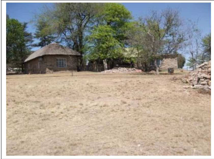
Figure 13- The main residence (FC02.1) (right) and an elongated outbuilding (FC02.1) which was constructed with the same material (left) (above). Note the dump with dresses and undressed dolerite stone suggesting that the complex of buildings was recently altered and upgraded (above).
