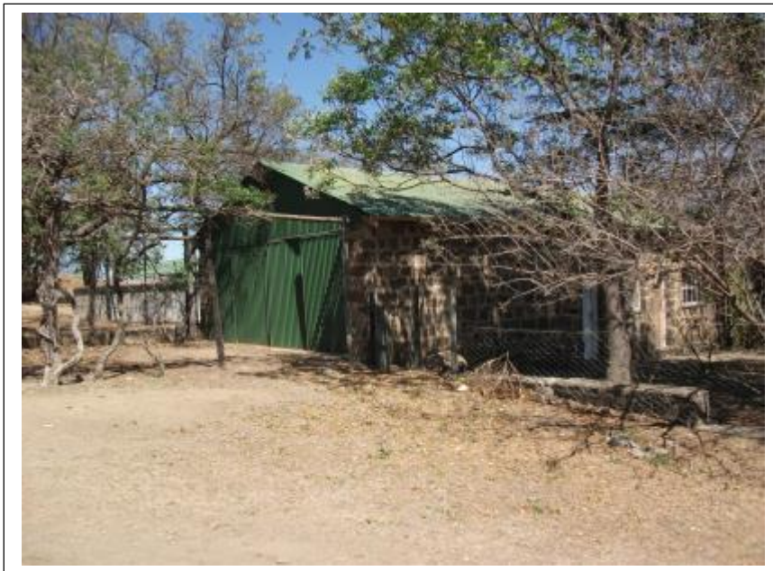
Figure 14- The second outbuildings in FC02 (FC02.1) has a near square ground plan and was constructed with dressed dolerite stone, fitted with steel window frames and steel door and is covered with a with pitched corrugated iron roof (above).
