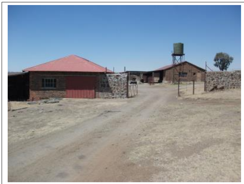
Figure 11- The two sheds (FC01.2, FC01.3) in FCO1 were both constructed with clay bricks and fitted with pitched corrugated iron roofs and steel window frames (above).
