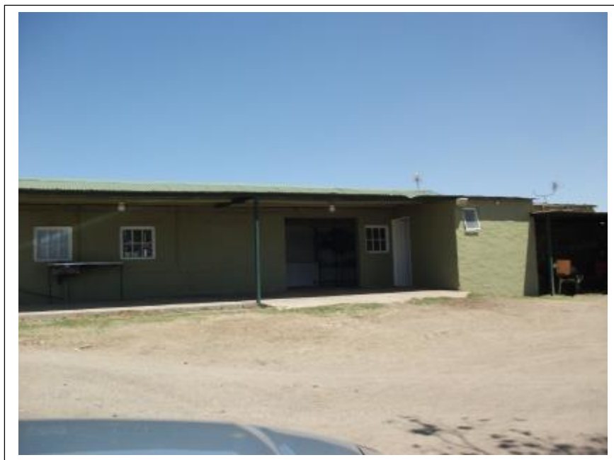
Figure 17- One of the extensions of FC02.5 was constructed with clay bricks and plastered with cement and is fitted with a low-pitched corrugated iron roof (above).
