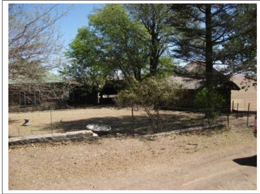
Figure 15- The rondavel (FC02.4) near the main residence. It was constructed with dolerite and fitted with a pitched grass roof (above).
