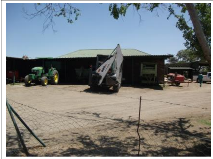
Figure 16- The shed complex (FC02.5) that is part of FC02 comprises several structures that were added to a main shed which was constructed with dolerite stone. The extended, plastered structures were constructed with clay bricks and perhaps with cement bricks as well. The fitted window and door frames were manufactured from steel (above).
