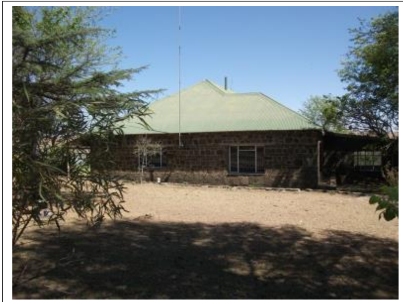
Figure 12- The main residence (FC02.1) in FCO2 was constructed with dressed dolerite stone and is a multi-roomed structure with steel window frames which was covered with a pitched corrugated iron roof (above).
