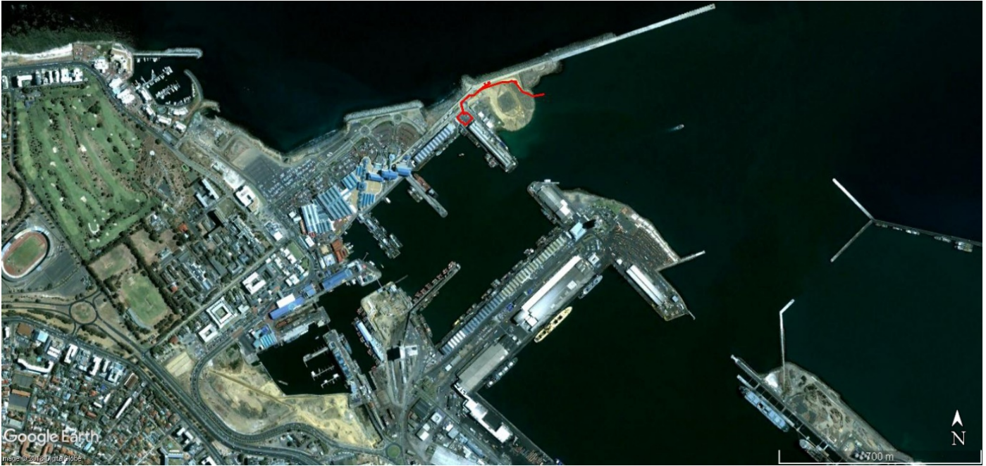
Figure 5.1.11: Proposed desalination plant infrastructure (red lines) indicated on 2000 Google Earth satellite imagery. The built footprint has increased significantly since 1993, and the Waterfront precinct now accommodates a number of hotels. The reclaimed area at the base of the breakwater to the east and north-east of the desalination plant site has been extended to its current extent, and all portions of the proposed desalination infrastructure located on land, are now located on land for the first time (Source: Chief Directorate National Geo-spatial Information).
