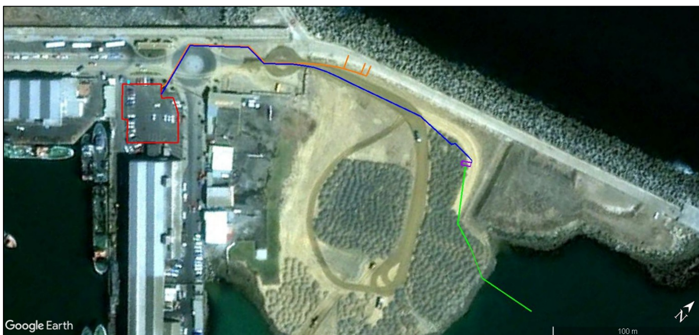
Figure 5.2.16: Detail of 2000-02-07 satellite imagery.
