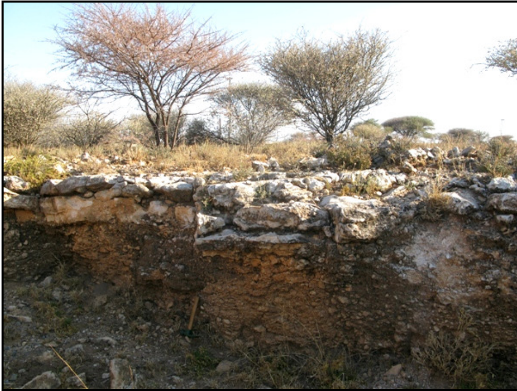
Fig. 21. Thick, nodular calcrete overlain by well-consolidated calcrete hardebank in a borrow pit just SE of the Herbert substation (Hammer = 27 cm) (Loc. 608).
