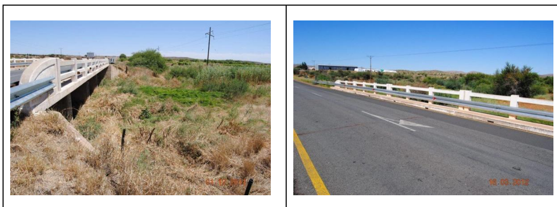
Fig. 5. Views of the bridge.
