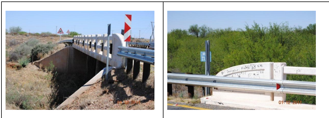
Fig. 2. Views of the bridge.
