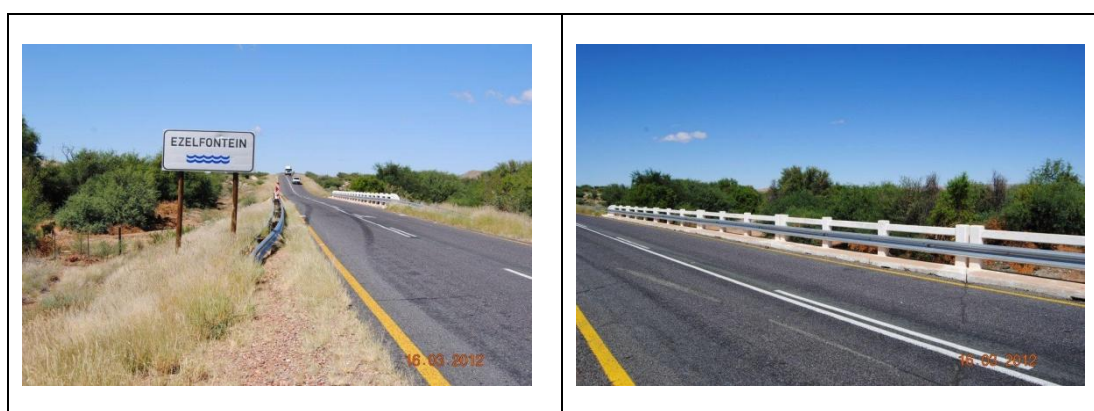
Fig. 4. Views of the bridge.
