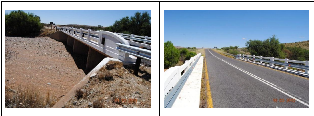
Fig. 3. Views of the bridge.
