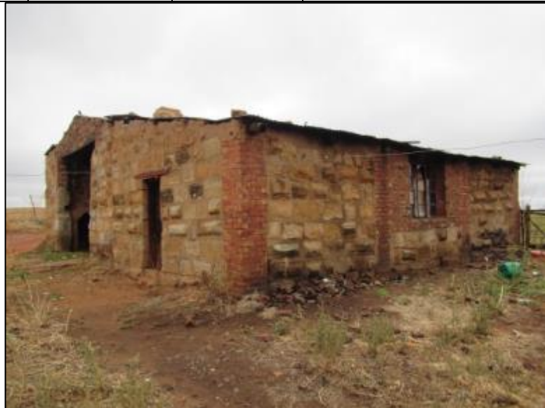
Figure 28 – View of the structure at KAL004
