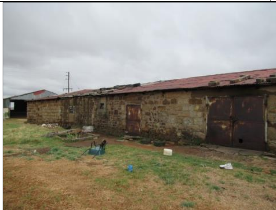
Figure 30 – View of the structure at KAL005
