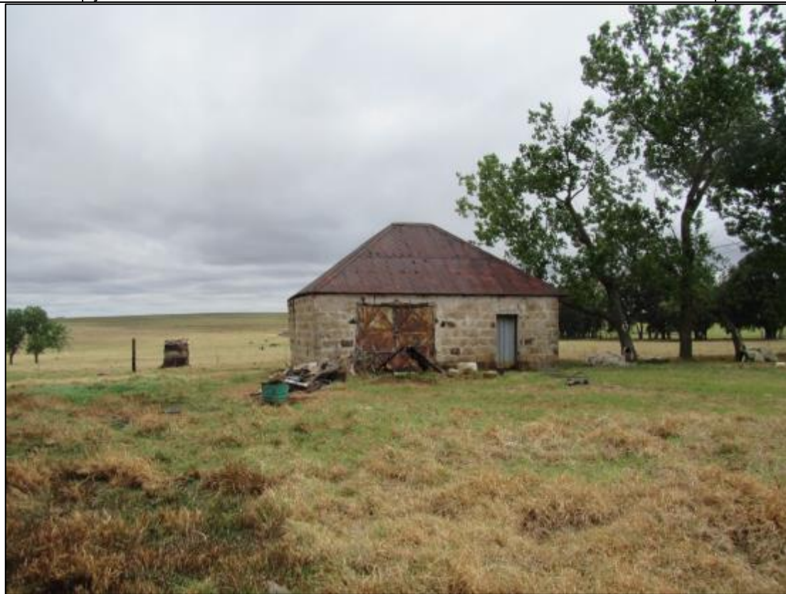
Figure 31 – View of the structure at KAL005
