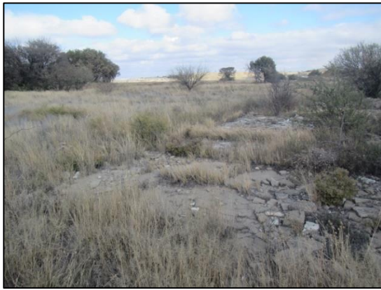
Figure 14 – Foundations of demolished buildings
