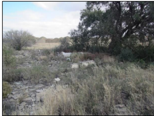
Figure 15 – Remains of demolished buildings at Site 211
