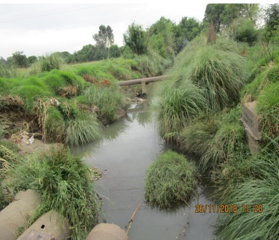
Photo 5: Existing 300mm Asbestos Pipeline
