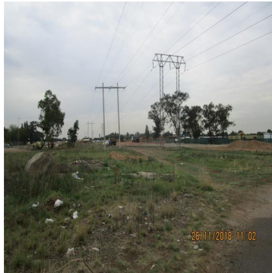
Photo 4: Existing overhead powerlines on site
