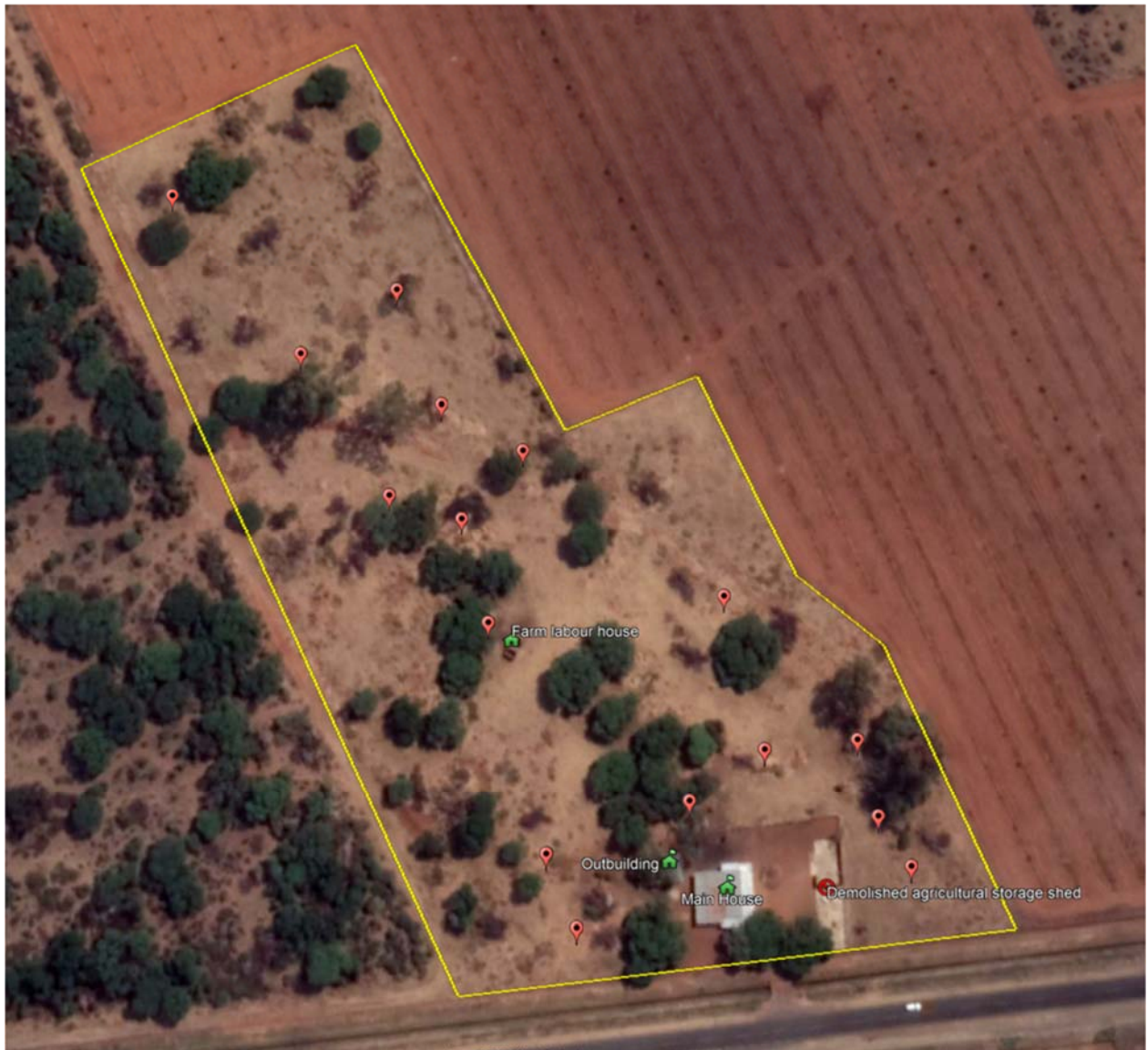
Figure 14: red balloons = dumping sites (building rubble, heaps of stones cleared from the surface areas, and mounds of soil); 3 existing buildings and the foundation of one two-roomed large agricultural storage shed:
