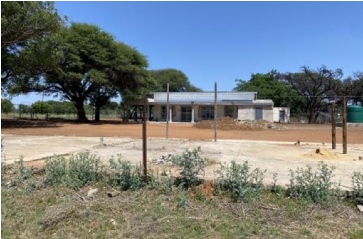
Figure 19: Eastern (and entrance side) façade of the farmhouse. Floor area of the demolished shed in the foreground. Note the dense vegetation at the bottom of the picture which is situated outside the cleared and fenced-in area. Building rubble of recent alterations to the house is visible in front of the house.
