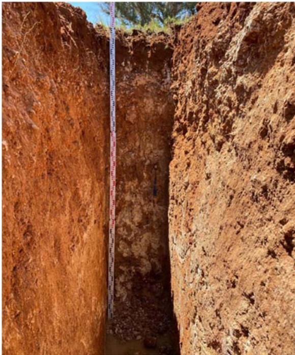
Figure 30: Walls of TP4
