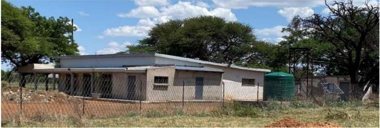
Figure 20: Eastern (left) and northern (right) facades of the main house showing recent additions of the verandah as well as the enclosed area at the northeastern corner.
