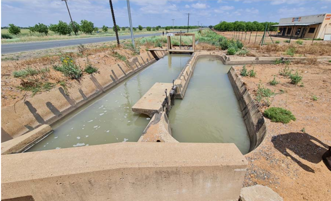
Figure 8: Example of a lot's feeding dam from a secondary canal
