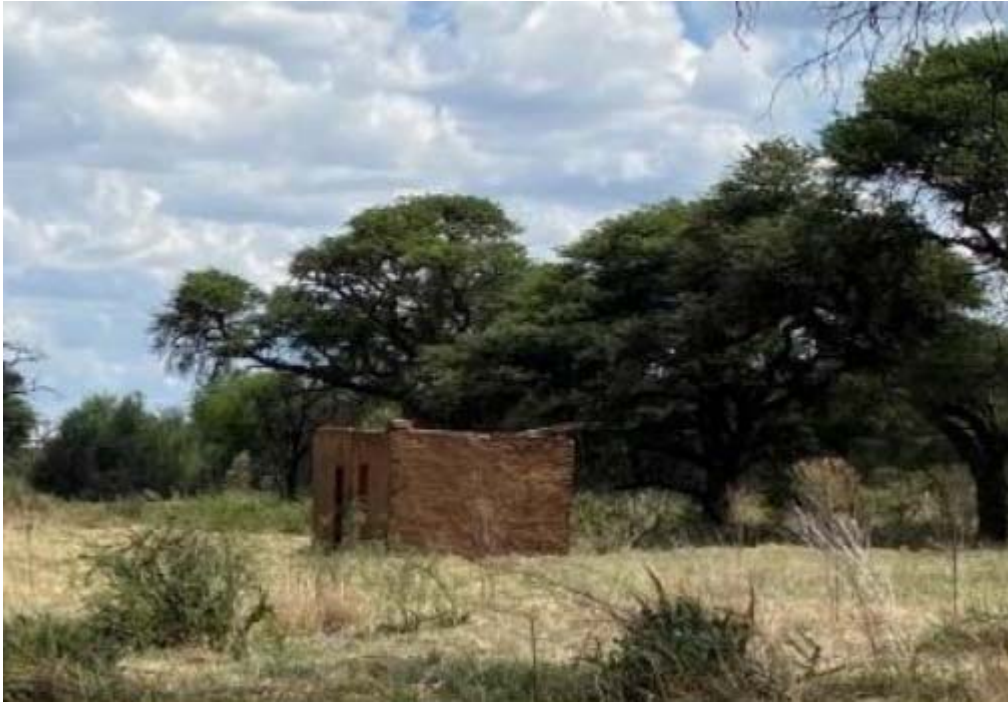
Figure 21: Labourer's house is a simple one-room flat-roofed structure of 5.5 X 4.5 m with a door and one window at its entrance facing north-west, situated approximately 9.5 m north-west of the main building.
