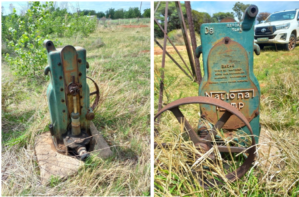
Figure 28: Close-up views back and front of the pump
