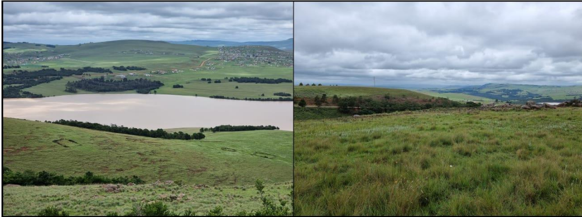
Figure 3-3: View of the Tsojana Dam and its surroundings in the larger project landscape.
