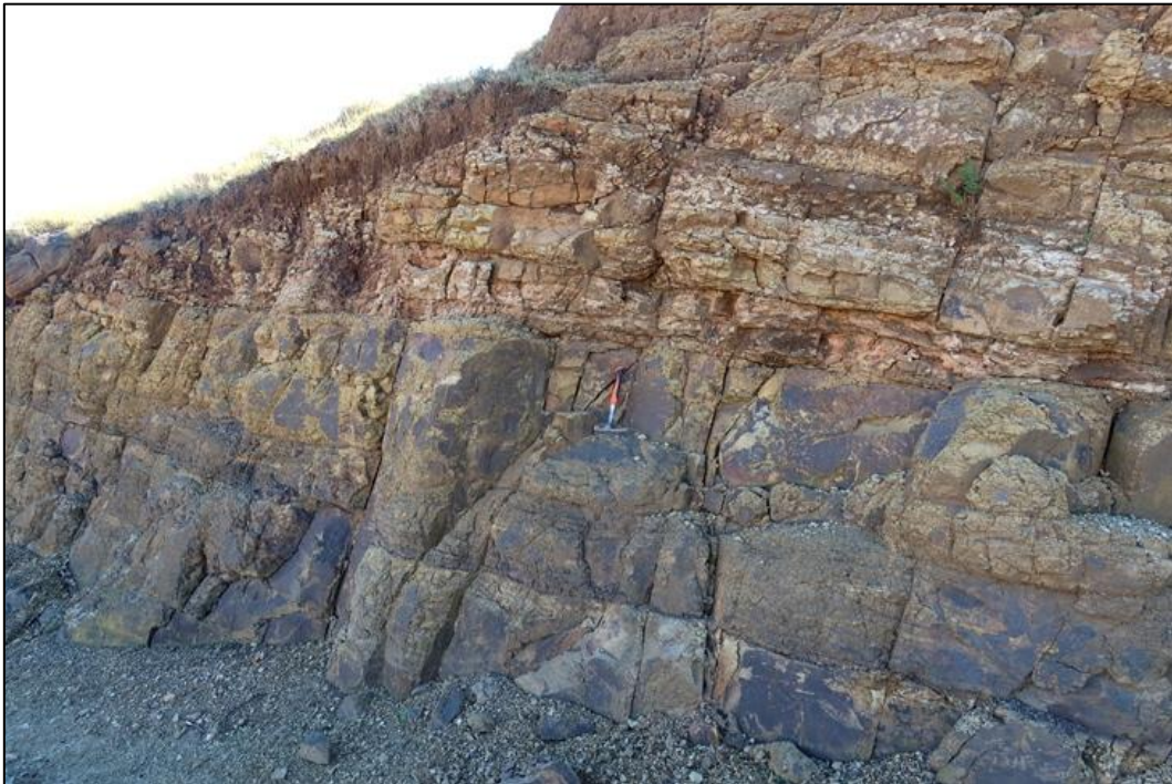
Figure 12: Deeply-weathered, mottled Burgersdorp Formation channel wackes (above) and grey-green to khaki overbank mudrocks (below) exposed in a road cutting towards the SW edge of the WEF project area on Farm RE/101 (hammer = 30 cm).
