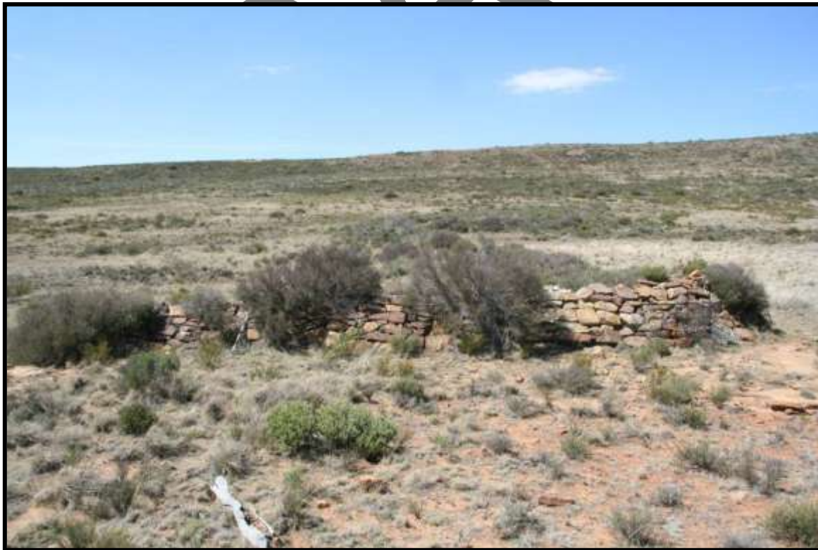
FIG. 11: SUPPORTING DAM WALL AT UMZ011
