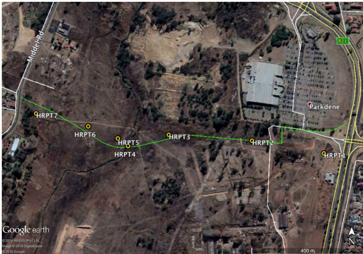
Figure 3.1 Satellite image of site showing the locality of the excavated trial pits.
