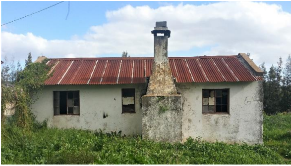
External chimney at Slaley (MF).
