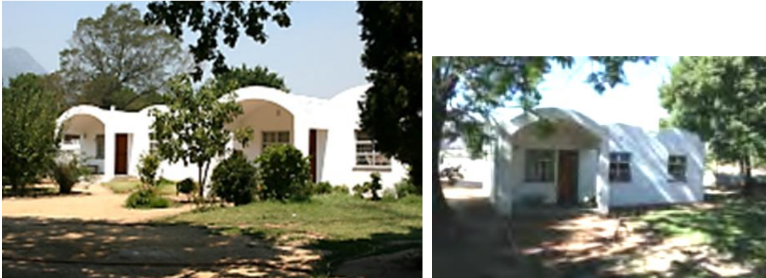
Workers' housing, Ida's Valley, designed by Gawie Fagan in 1975 (Barker 2012).
