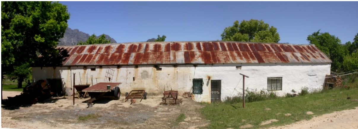
Corrugated-iron roof with raised eaves on an outbuilding at La Cotte, Franschhoek (AM 2007).
