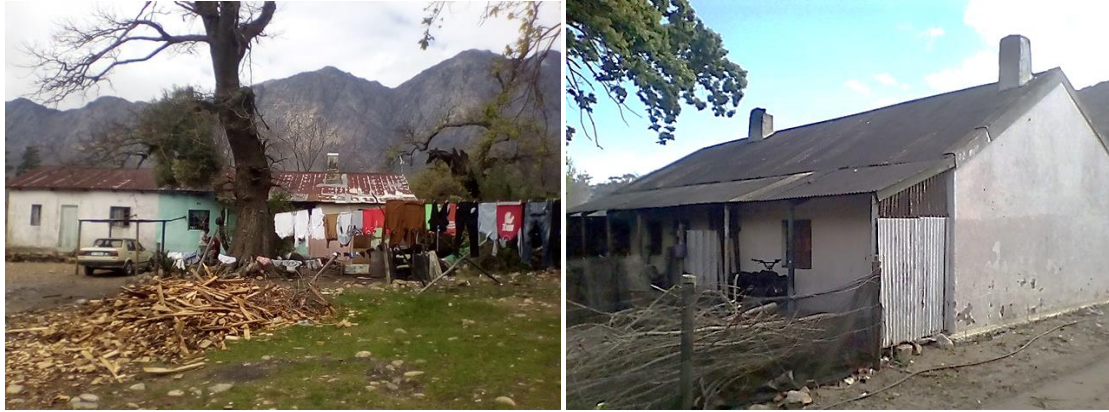
Clusters of buildings in poor condition, on Le Franschoek and La Provence (Die Vlei) (FT).
