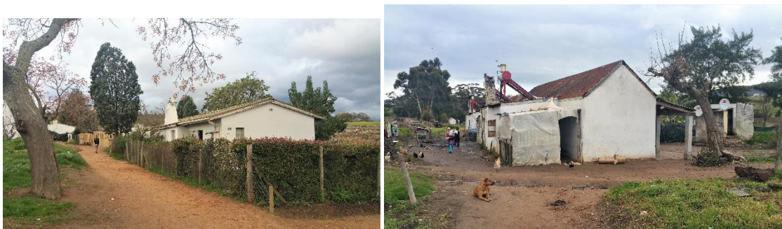
Free-standing cottages and rows of rooms in Devon Valley (MF 2017).
