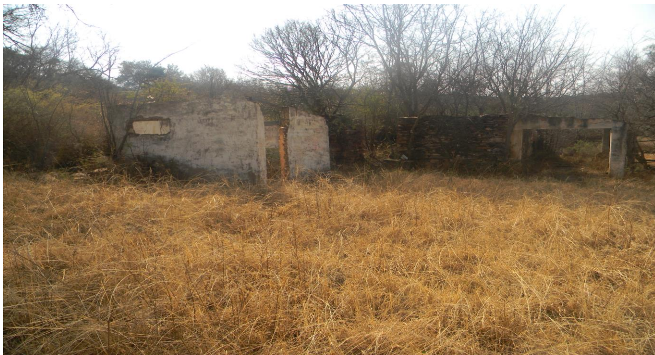
Plate 31: Photo 31: View of abandoned farm house and structures on the bank of the Blaauwbank River (Photograph © by Author 2018)
