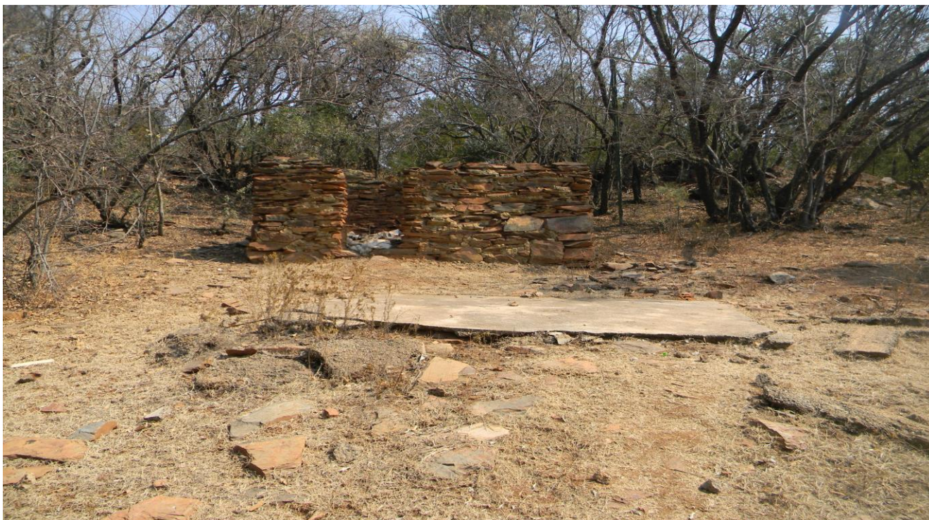
Plate 41: Photo 41: View of recent stone and mud house with cement floors (Photograph © by Author 2018)
