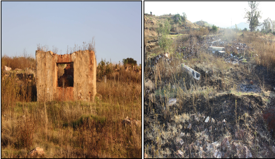
Figure 5: View of a stone constructed building and farm house foundation on the right
