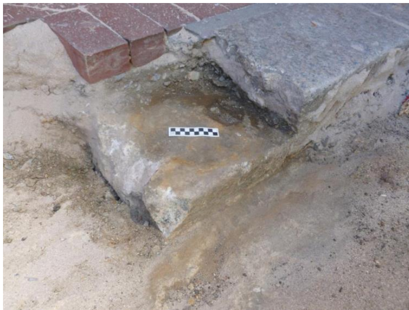
Figure 21: Sandstone foundation slab for granite kerbing
