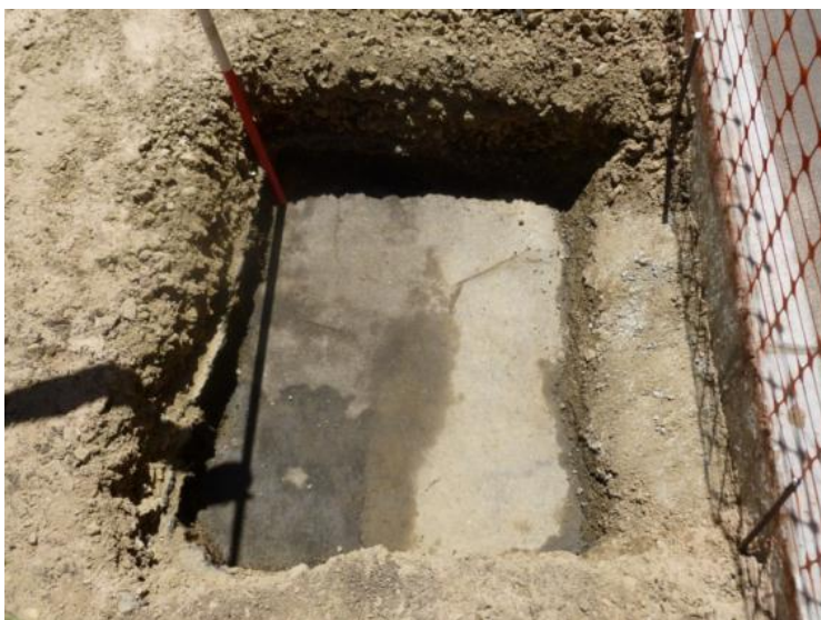
Figure 7: Cemented foundation level after removal of wooden cobbles
