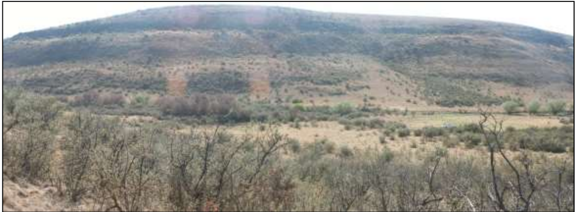
Fig. 4 Proposed dam-wall site from the west.
