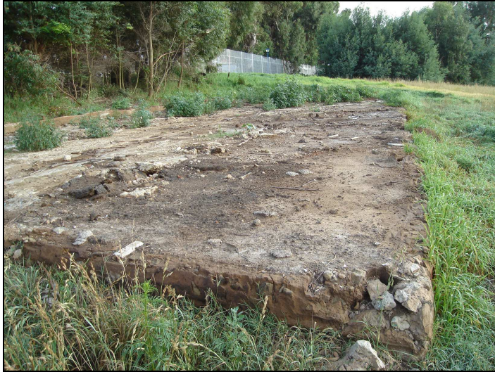
Fig.21 The foundation and floor of the old shed after demolition.
