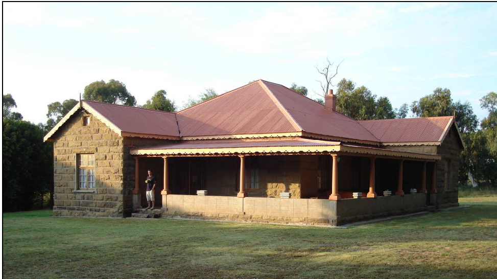
Fig.12 Sandstone house is presently being used as visitors' accommodation.
