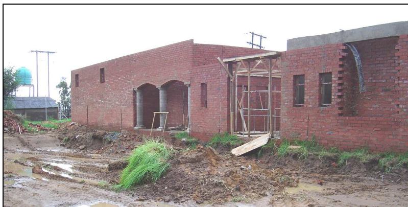
Fig.19 New SAPD buildings under construction.
