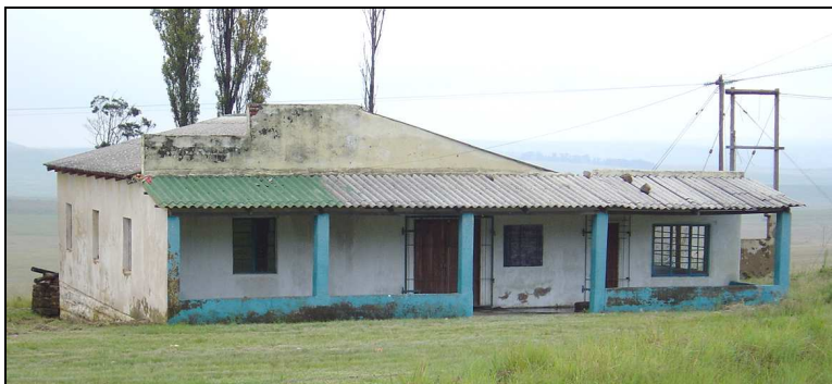
Fig.14 One of several old houses at Verkykerskop.
