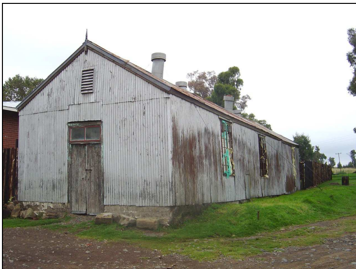
Fig.7 Front view of the old mill building.
