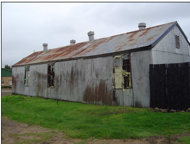
Fig.8 Rear view of the old mill building.
