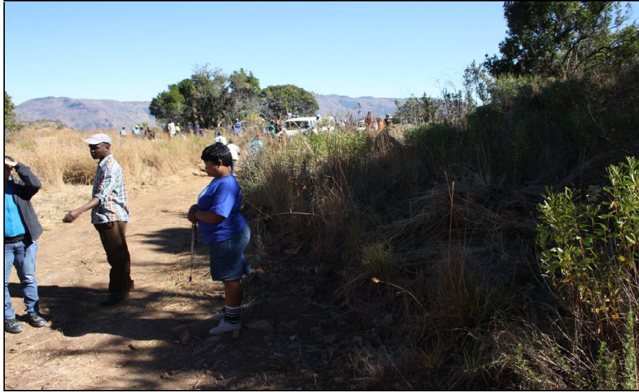
Figure 1: View of the disturbed site with community members standing in the middle of the newly constructed gravel access road across the affected stone wall enclosure site
