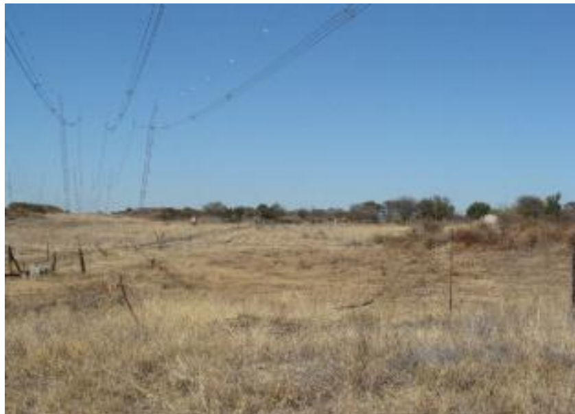
Figure 2: One view of section of area next to existing line.
