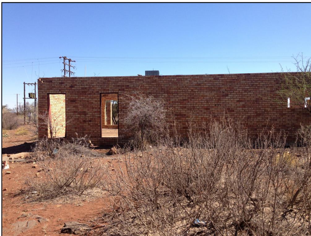
Figure 7: Recent structure on the study area viewed from the southeast (Col 1)
