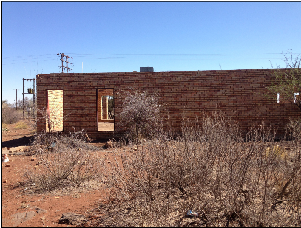
Figure 10: Recent structure on the study area viewed from the southeast (Col 1)
