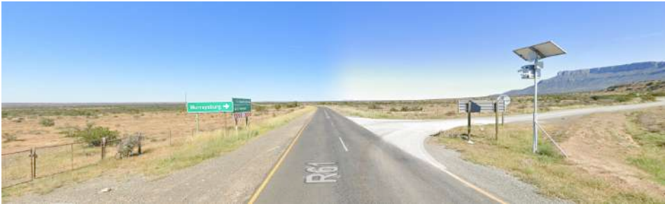
B. Streetview: R61 intersection with secondary, gravel road to Murraysburg
