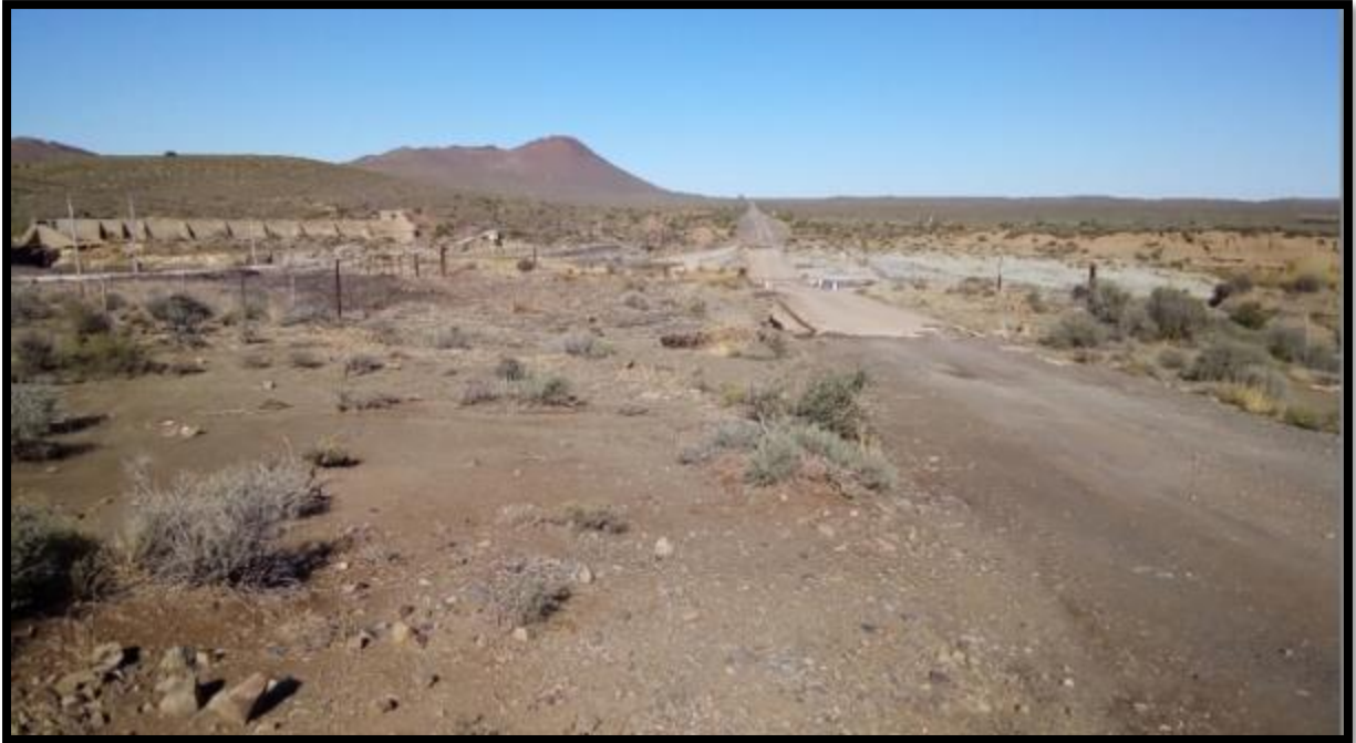
Figure 19: Low water crossing over Sakrivier. Poorly sorted scattered dolerite, sandstone and hornfels are present as well as unconsolidated gravely Cenozoic superficial deposits.
