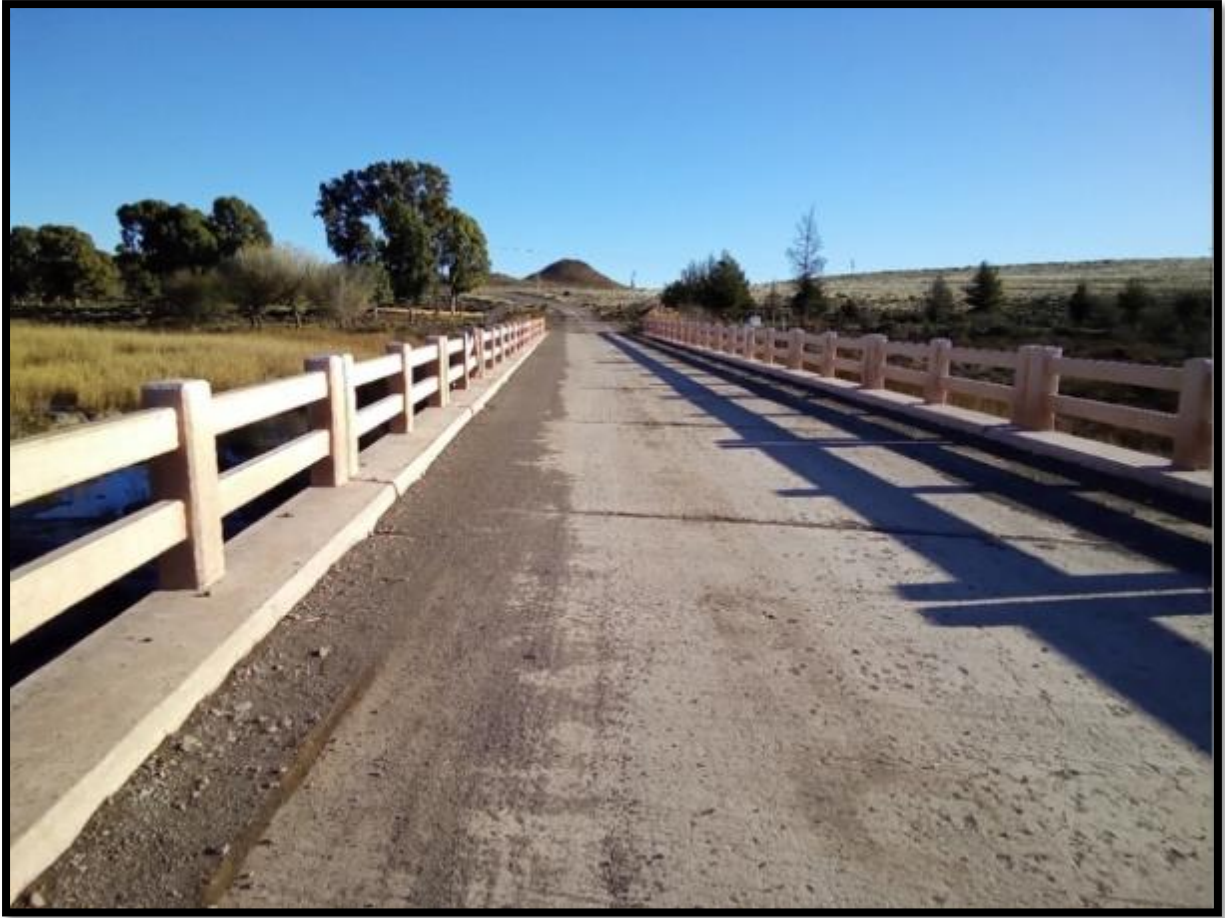
Figure 29: Concrete bridge built in 1952.
