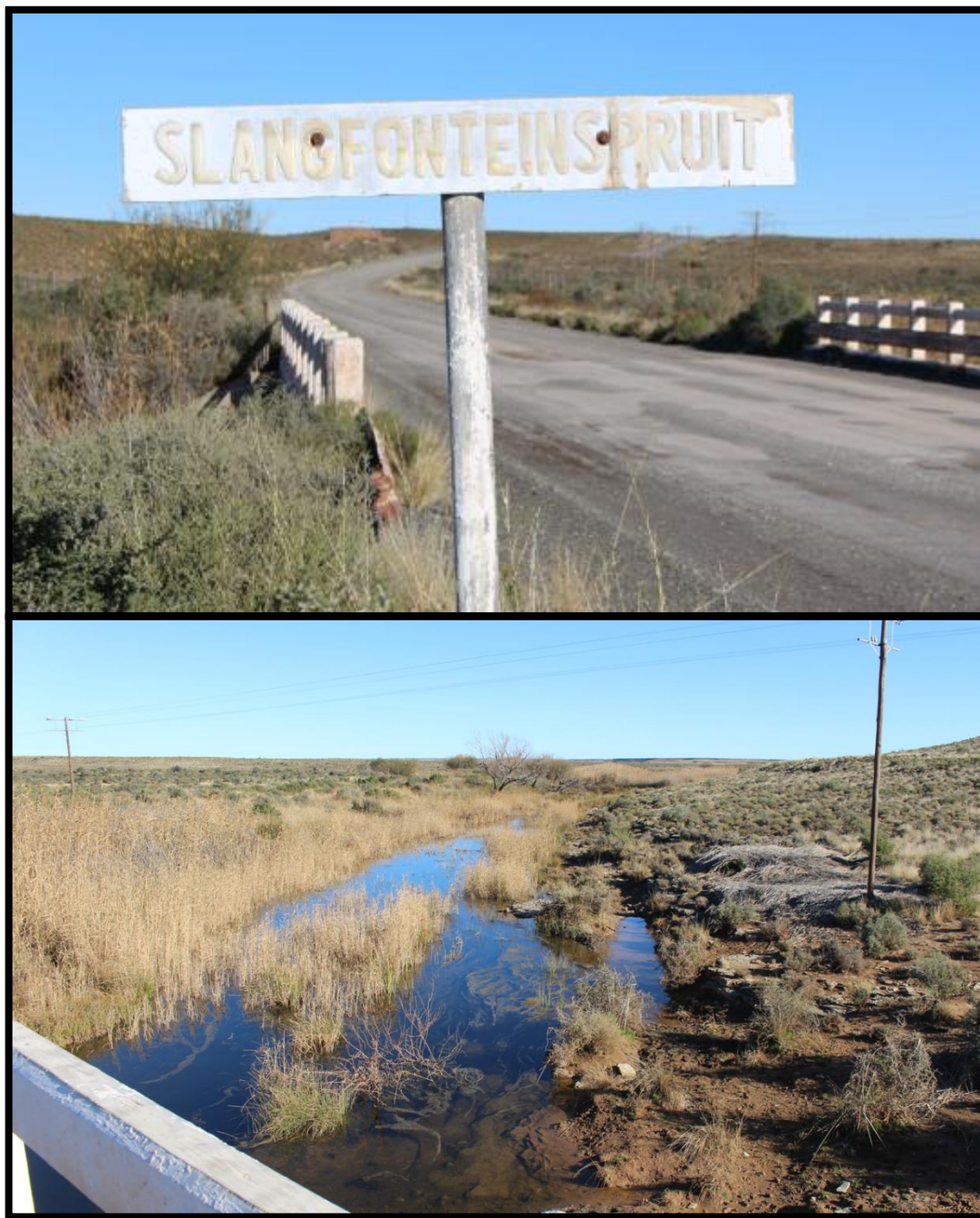
Figure 35: Slangfonteinspruit comprises of sand with isolated mudrock outcrops and thick vegetation.
