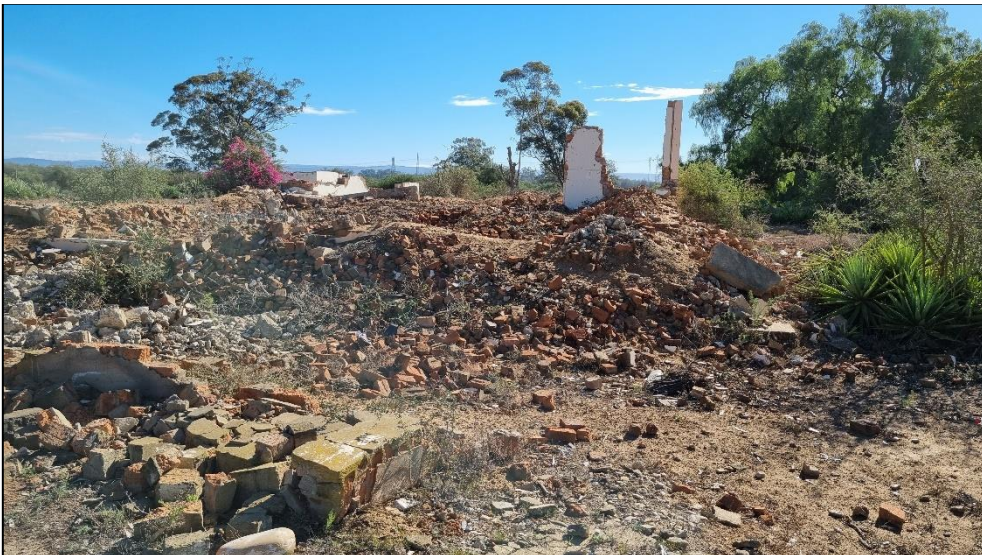
Figure 26. View of the of the remains of the school buildings.
