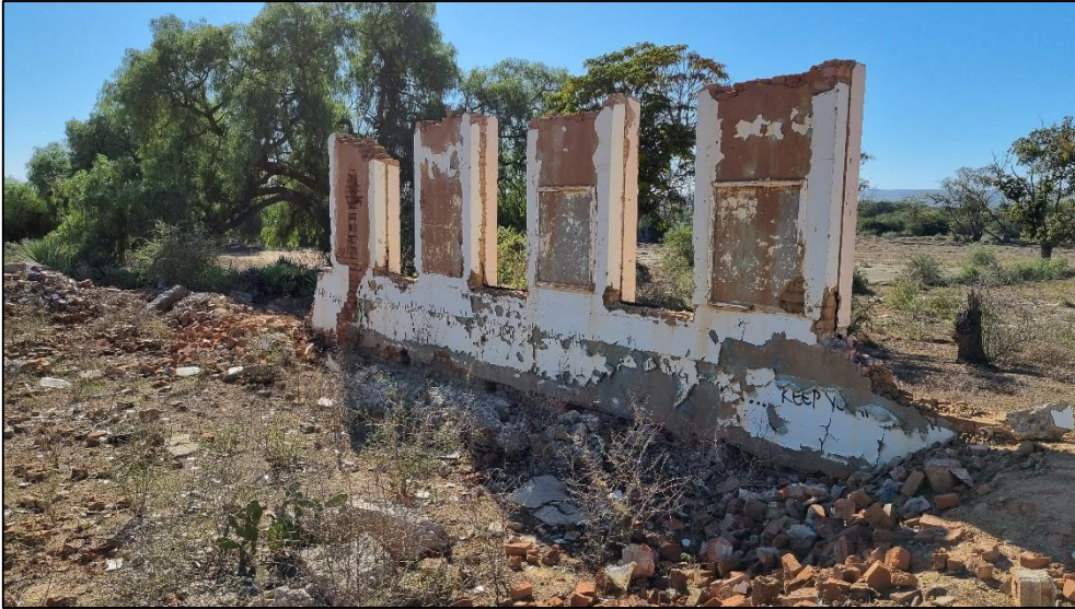
Figure 25. View of the of the remains of the school buildings.
