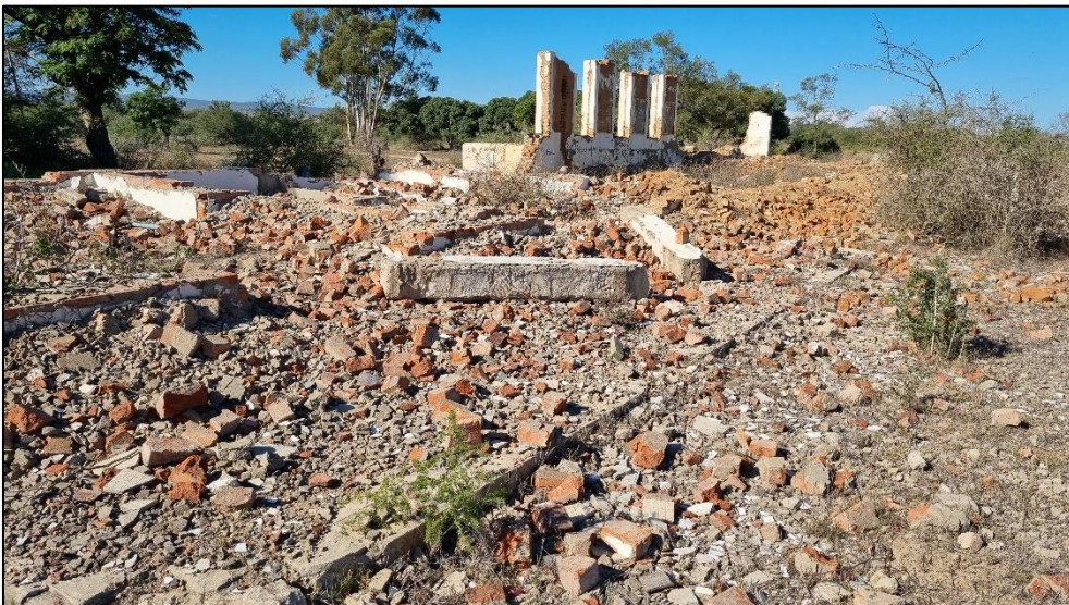
Figure 24. View of the of the remains of the school buildings.
