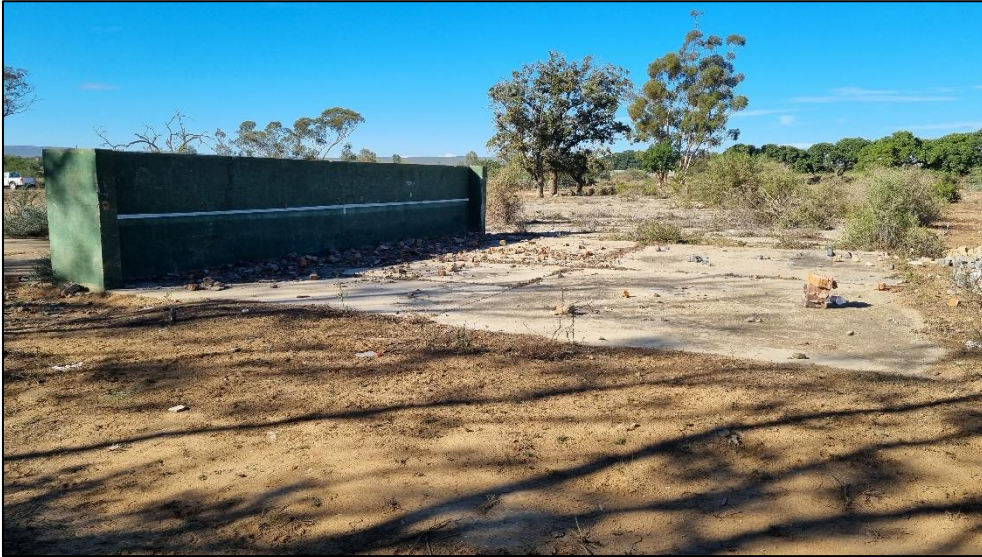
Figure 22. View of the of the remains of the school associated infrastructure.
