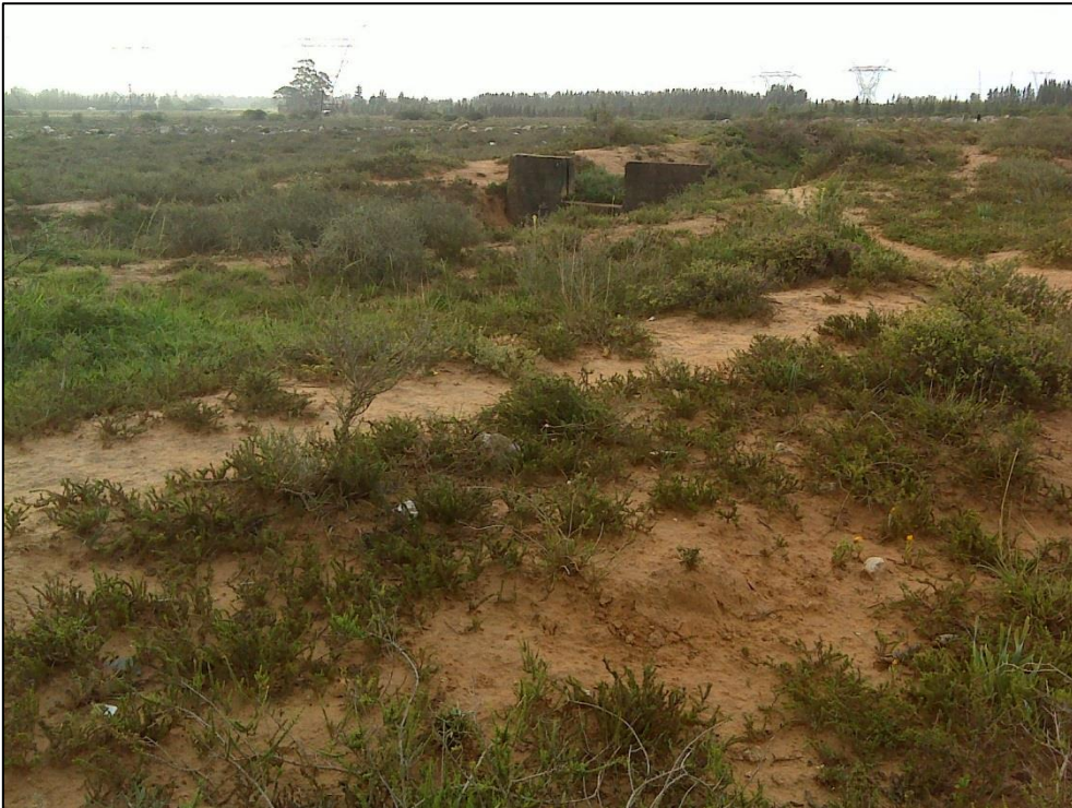
Figure 17. Example of retaining walls / weirs located along the proposed pipeline route.
