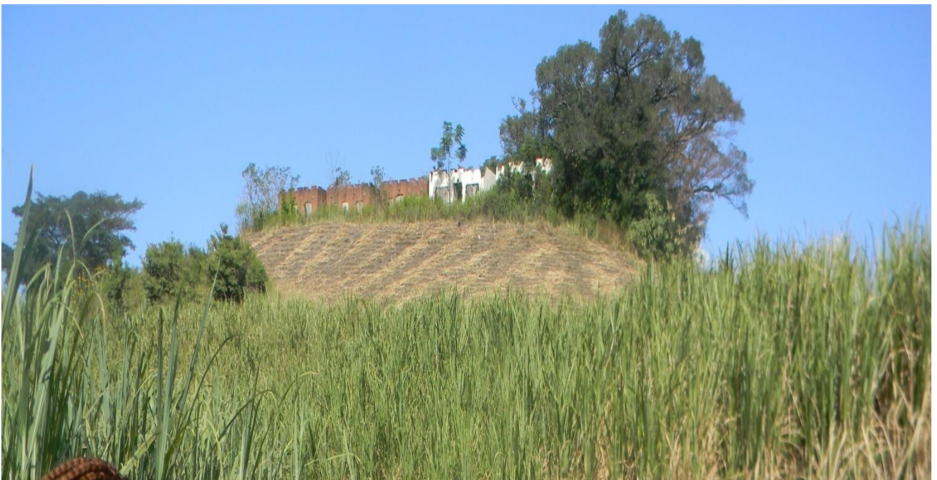
Plate 33: showing old buildings located within the proposed pit site.(Cluster 2)
