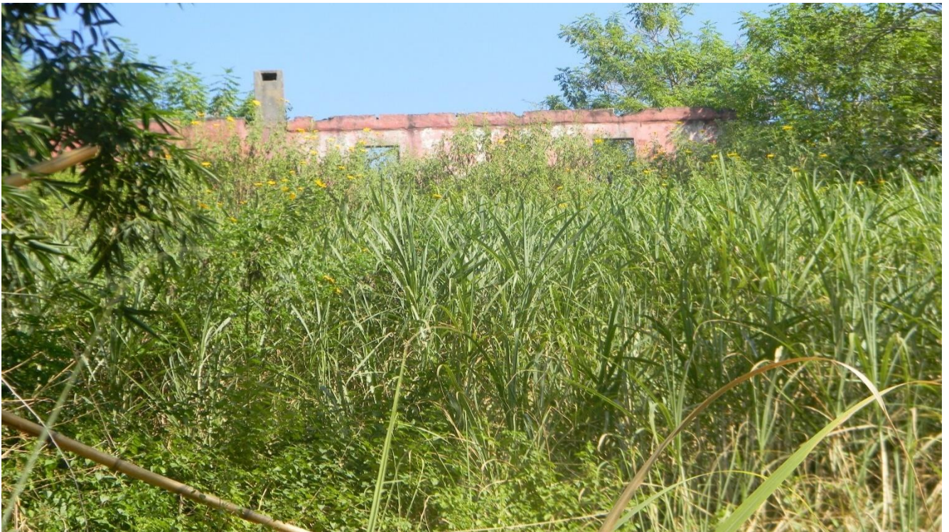
Plate 31: showing old buildings located within the proposed pit site (Cluster 4).
