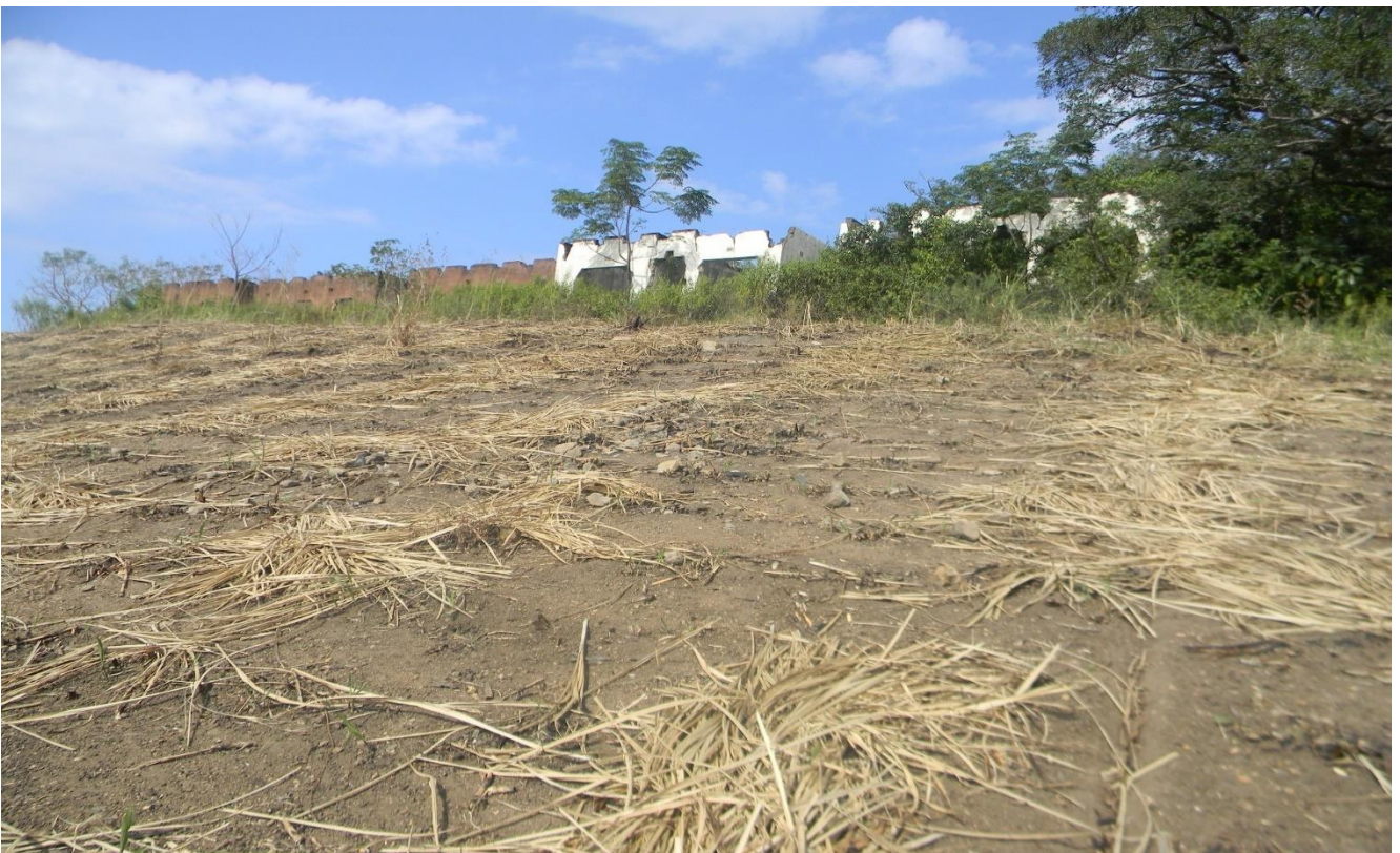
Plate 27: showing old buildings located within the proposed pit site (Cluster 2)
