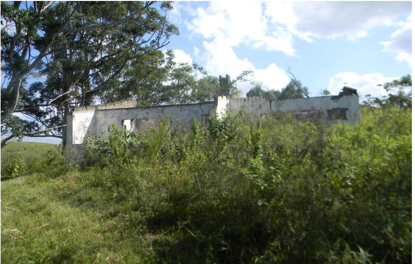
Plate 30: showing old buildings located within the proposed pit site (Cluster 3).
