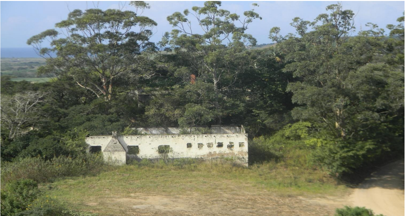
Plate 26: showing old buildings located within the proposed pit site.
