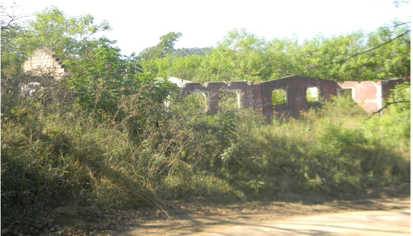
Plate 32: showing old buildings located within the proposed pit site (Cluster 4).
