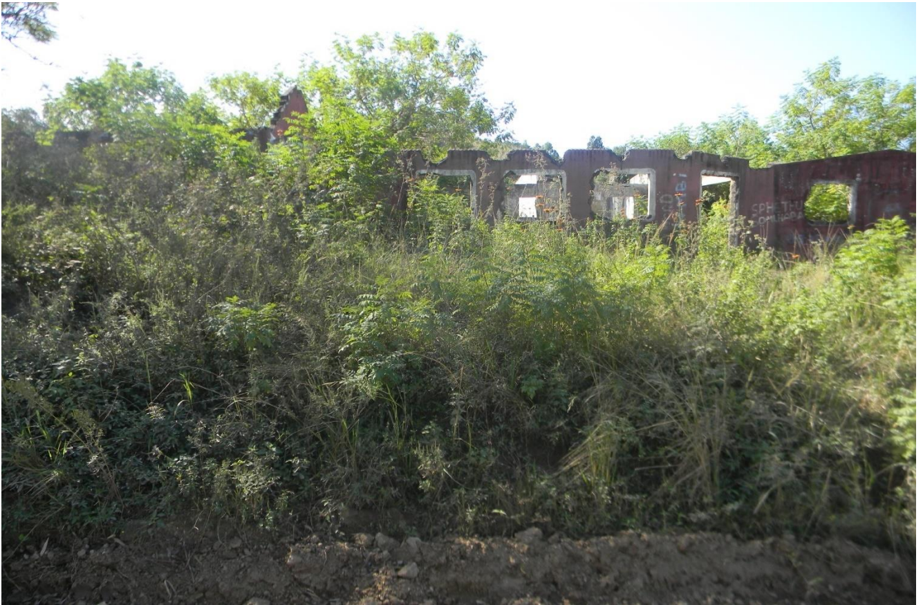
Plate 34: showing old buildings located within the proposed pit site (Cluster 4).
