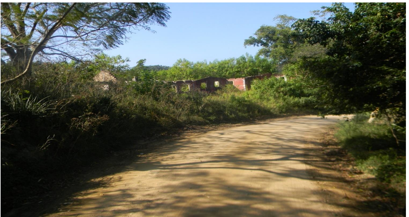
Plate 35: showing old buildings located within the proposed pit site (Cluster 4).
