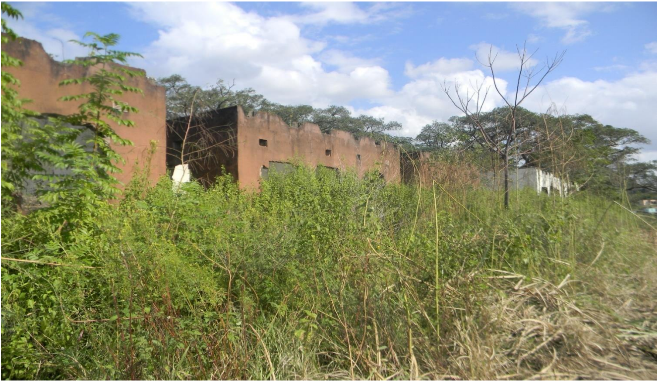
Plate 28: showing old buildings located within the proposed pit site (Cluster 2).
