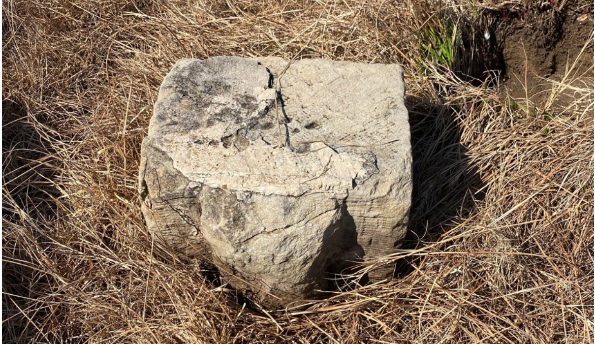
Figure 25. Example of a dressed piece of sandstone area (approximately 380mm x 380mm x 300 mm). Several of these pillar blocks and also the blocks of a sandstone arch are scattered over a large.
