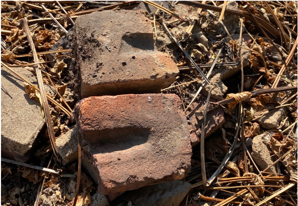
Figure 25. Example of a dressed piece of sandstone area (approximately 380mm x 380mm x 300 mm). Several of these pillar blocks and also the blocks of a sandstone arch are scattered over a large.
