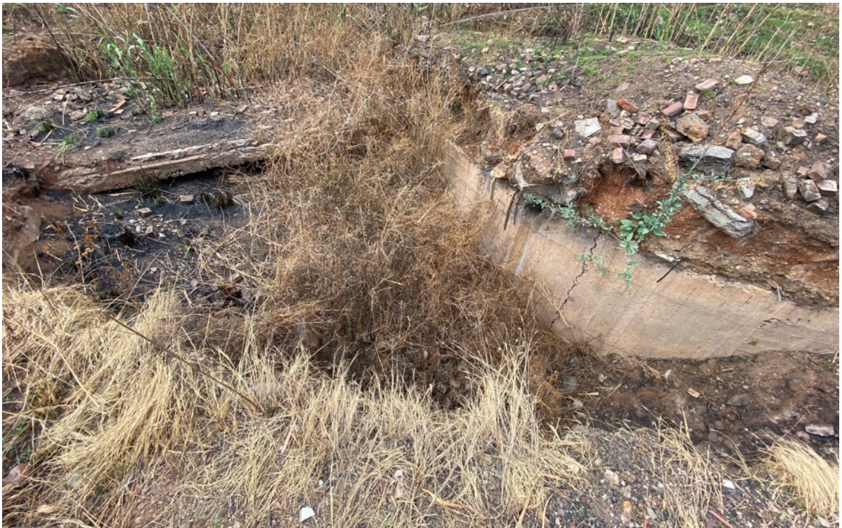
Figure 11. Remains of former mining infrastructure in the south-eastern corner of the site.
