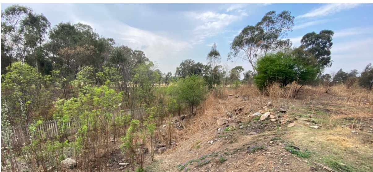
Figure 9. Extent of fill along the boundary with the golf course.
