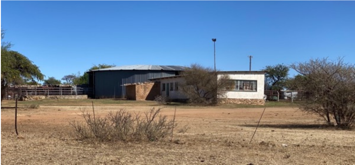
Figure 7. Modern buildings associated with animal handling and care.
