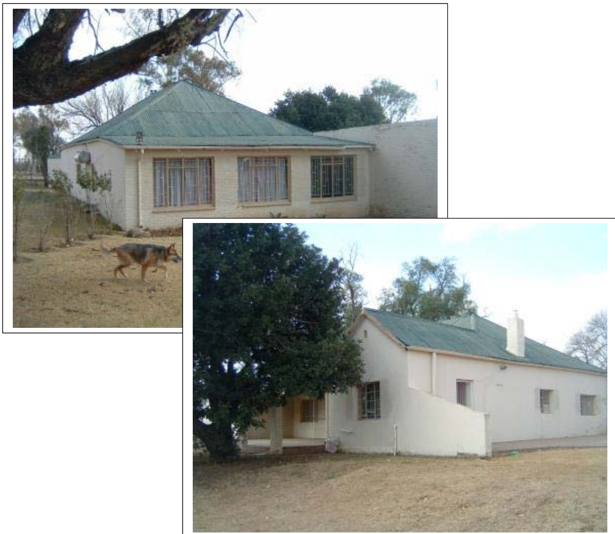
Figure 9 & 10- Historical House 01 is a square structure which was constructed with sandstone and cement. It is fitted with a pitched corrugated iron roof (above).
