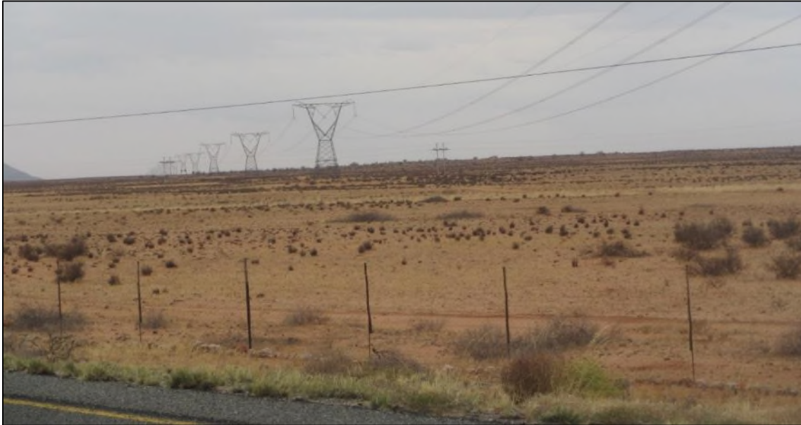
Figure 4: View towards the east along the Alternative 1 corridor showing the existing 400kV power line that it follows.
