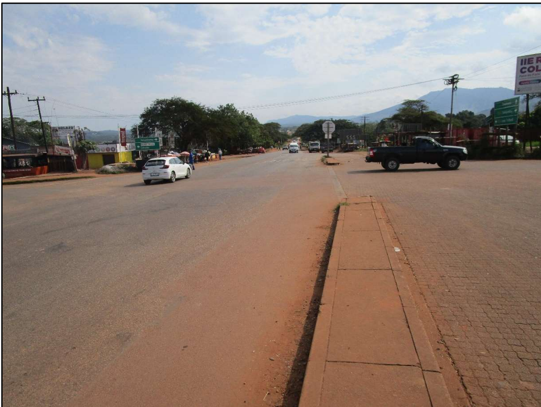
Figure 14. A roadside view at position 8 on figure 4 within Tshakhuma – westerly direction.
