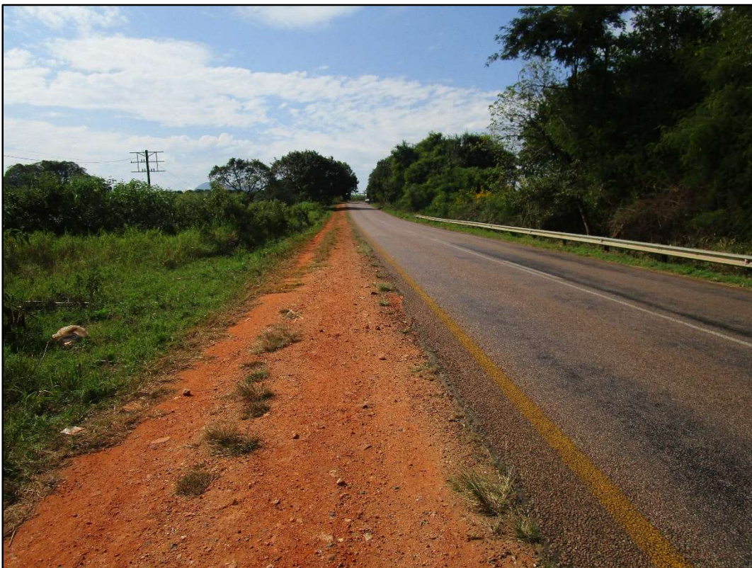
Figure 10. A roadside view at position 5 on figure 4 – easterly direction.
