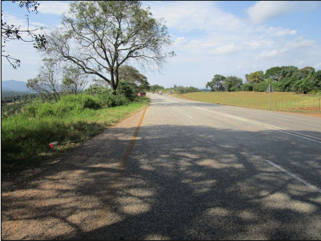
Figure 11. A roadside view at position 6 on figure 4 – easterly direction.
