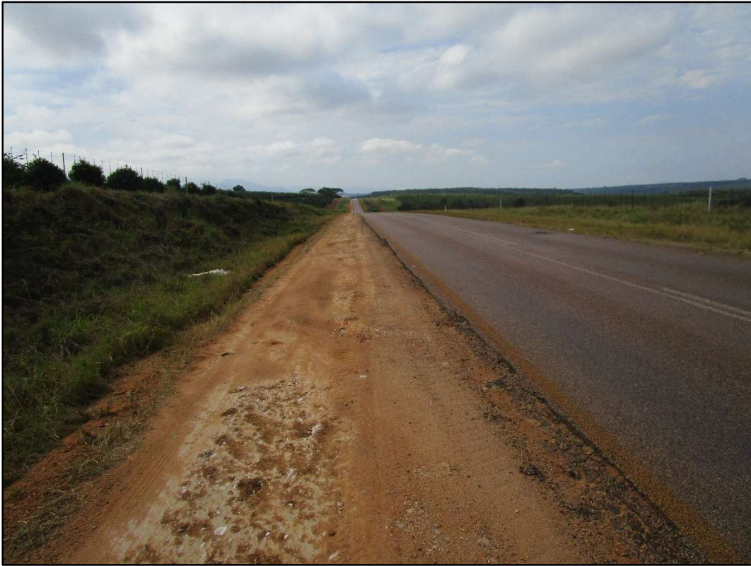
Figure 7. A roadside view at position 2 on figure 4 – easterly direction.
