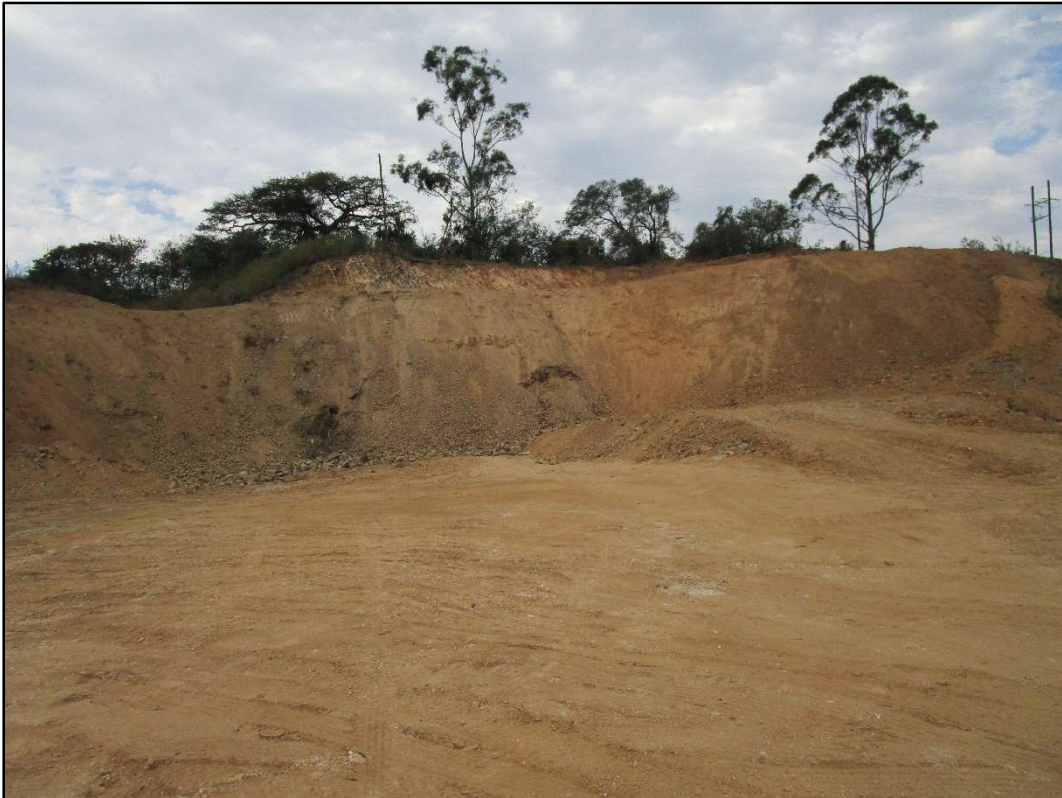
Figure 15. A view of the borrow pit at 16.8 km along the R524.
