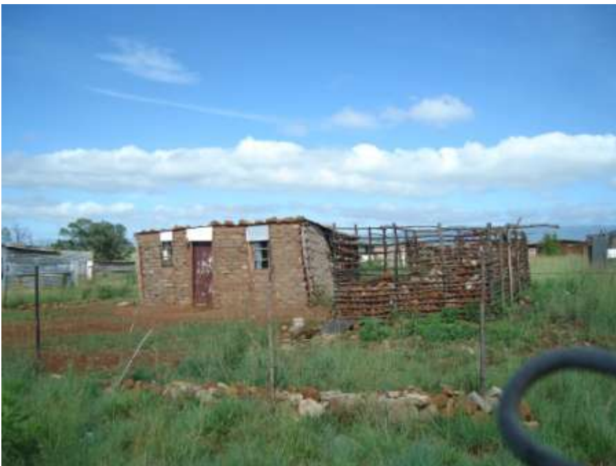
Typical shack, Siyahlala-La. S 27° 46' 45,5" and E 29° 55' 44,8".
