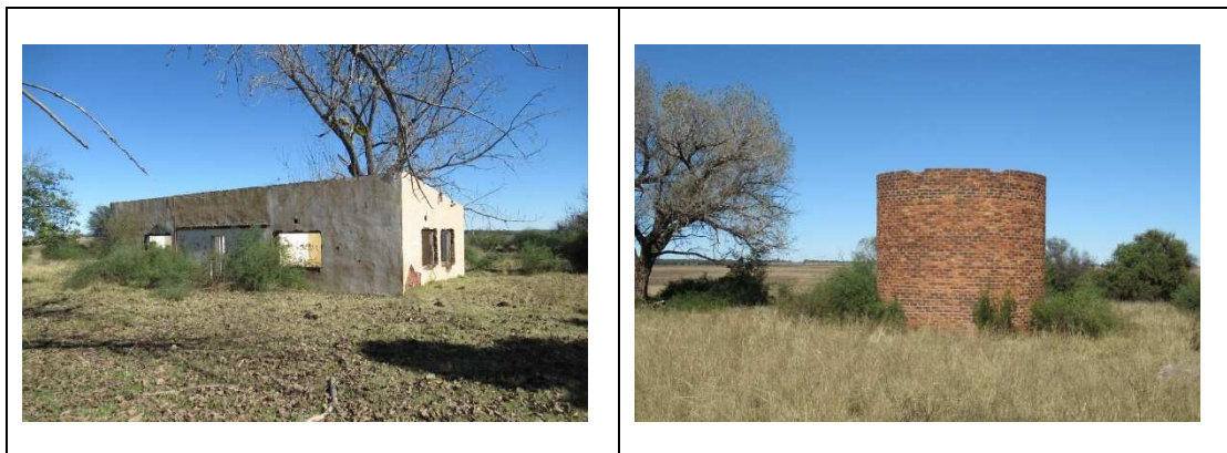
Figure 13. Remains of the "Groenfontein" farmstead
