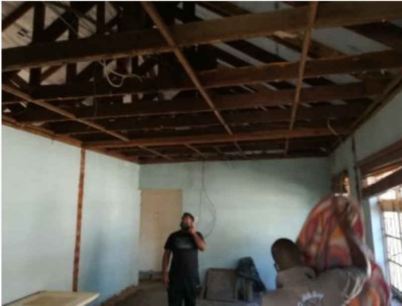
4. Internal Main Dwelling (Roof Structure rot and Borer infestation)
