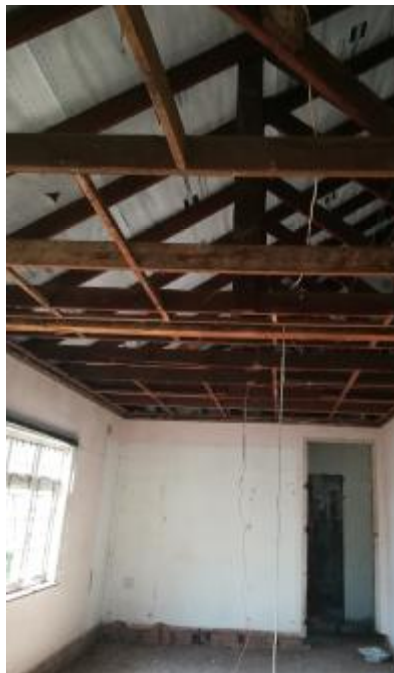
4. Internal Main Dwelling (Roof Structure rot and Borer infestation)
