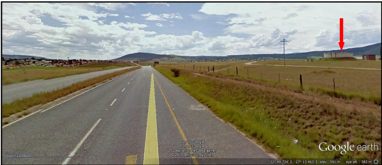
Plate 5: View in a westerly direction along the R63, towards Debe Nek. The reservoir (R1) marked with a red arrow will be replaced with a larger reservoir. The pipeline will follow the R63 and will be placed in the road reserve.
