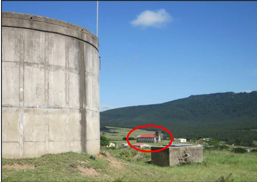
Plate 9: The reservoir (R5) which will be ungraded in the foreground, and the Bryce Ross Memorial Church in the background (circled in red).
