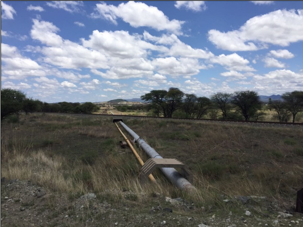
Figure 9. High pressure air line on the site
