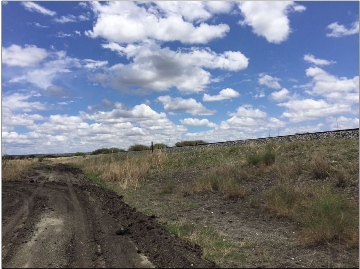
Figure 10. Current railway embankment on the site
