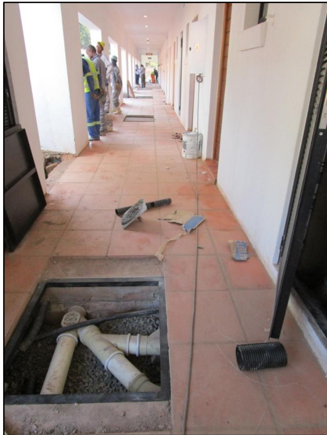
Figure 10. View of new location of the services trench on the passage.
