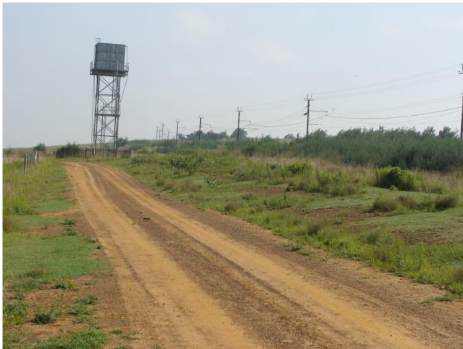
FIGURE 11: VIEW ALONG ONE OF THE WATERLINE ROUTE BETWEEN W1 AND W2.
