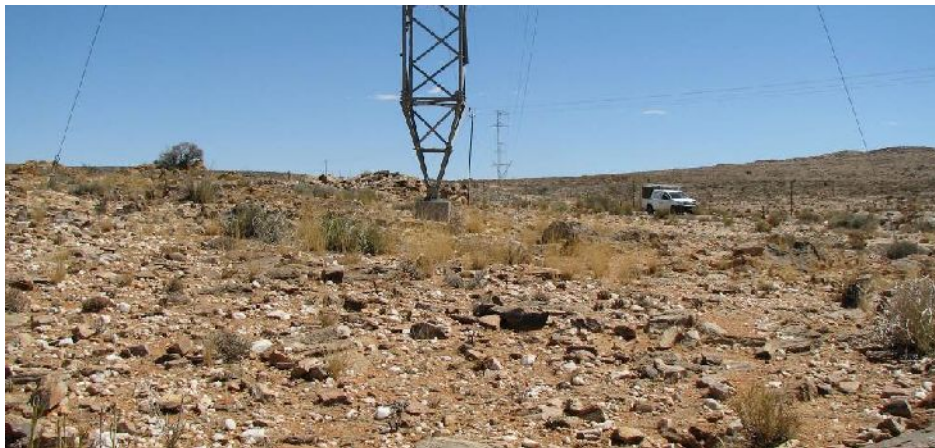
Figure 7. Minimal disturbance in the vicinity of a tower on an existing transmission line.
