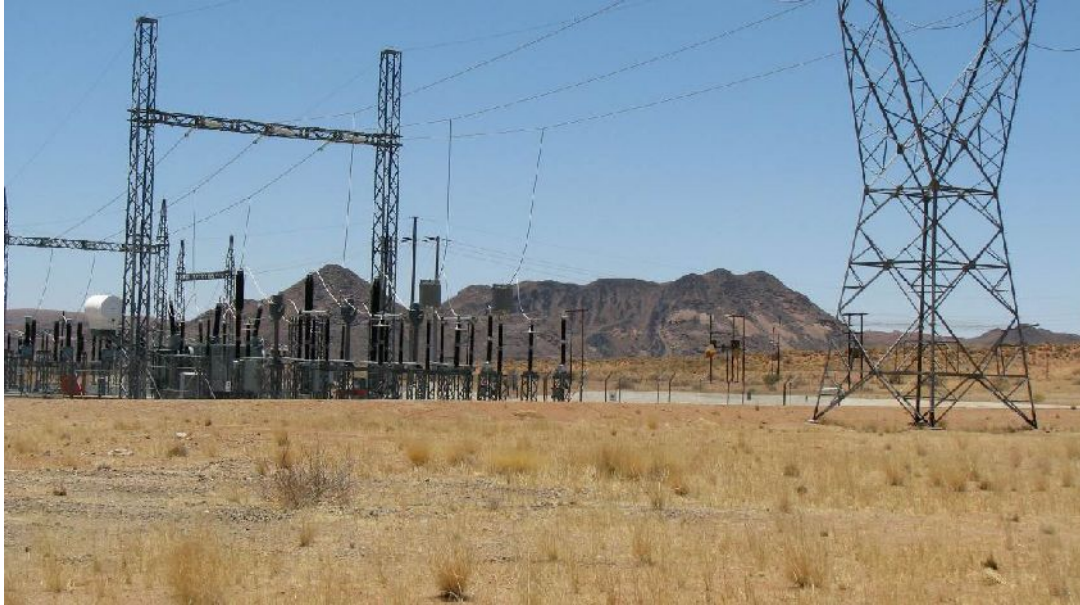
Figure 11. Already disturbed areas around the Paulputs Substation – no heritage traces found.
