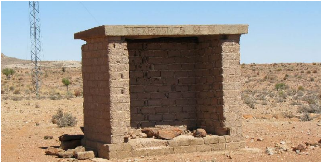
Figure 6. Remains of pre-1961 mining infrastructure.
