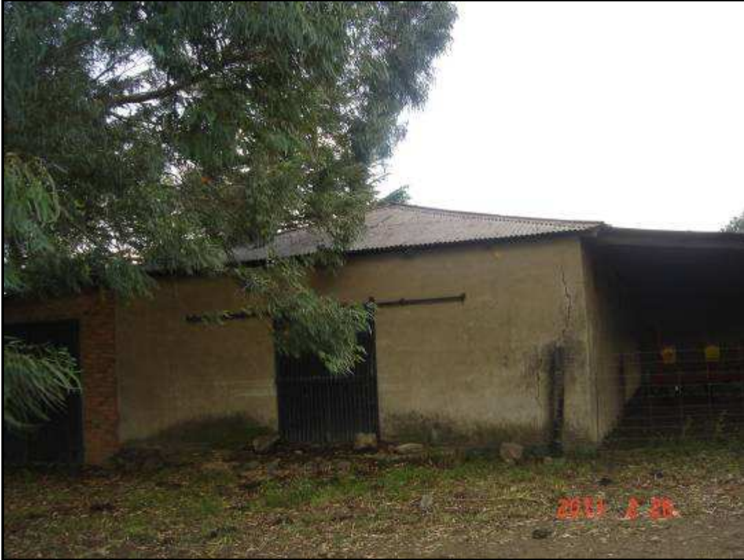
Plate 14: Structure A – Farm Buildings (Portion 61 of farm Enon 61HS)
